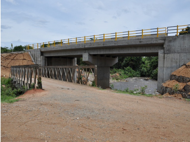
Double span Wambabya concrete 23.6m span girder bridge (right) replaces the steel Bailey Bridge (foreground).
