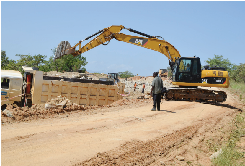
Section of Moroto-Nakapipirit road at Kamusalaba under construction
