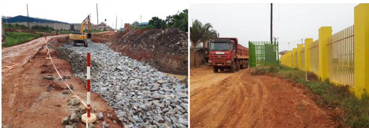
L-R: Ongoing civil works (rock filling), UMEME transformer erected in the road corridor at KIBP-Namanve
