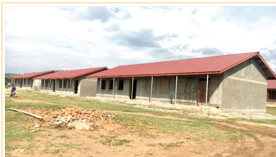
Construction of Bunambutye Seed Secondary School in Bulambuli District - Eastern Uganda
