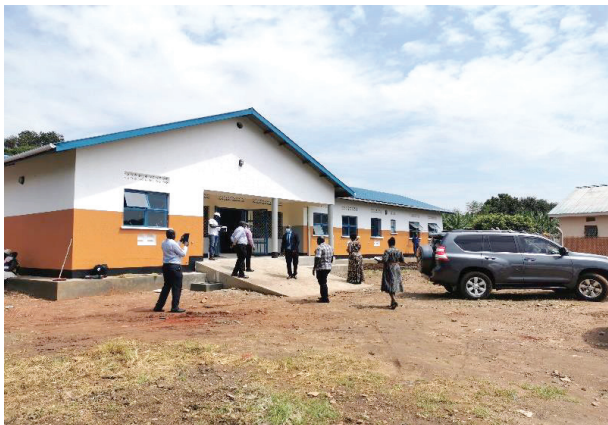
Front View of the completed Upgraded Pandwong HC III, Kitgum Municipal Council
