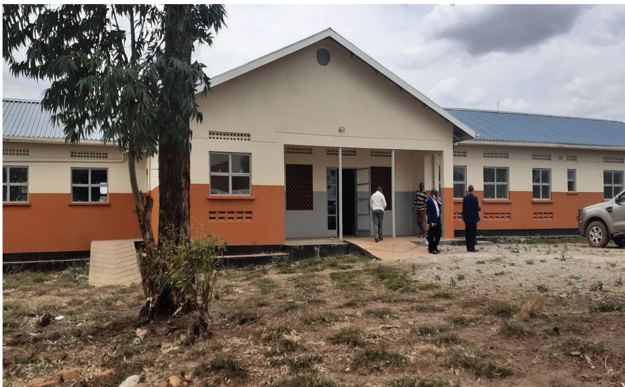
Completed New Maternity General Ward at Kaziba HC II in Gomba District, Central Uganda
