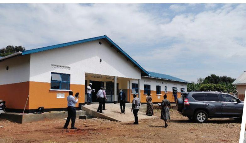
Front View of the completed Upgraded Pandwong HC III, Kitgum Municipal Council
