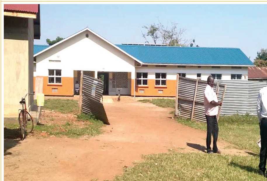
Completed General Maternity Ward at the upgraded Nawangisa HC II to III, Bugweri District, Eastern Uganda
