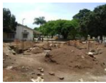
Excavation of information centre
