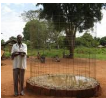
Construction of a water tank in a beneficiary's home, Kamuli district
