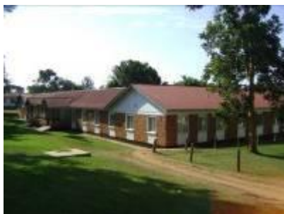
Rehabilitated interns' hostel
