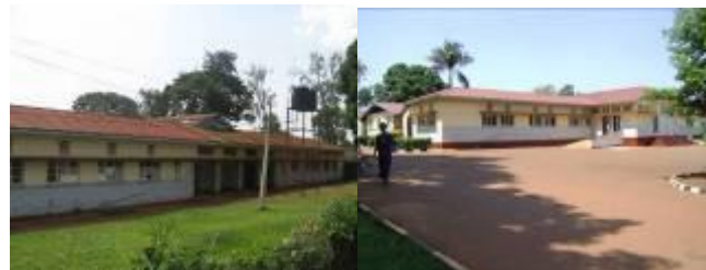
OPD before and after renovation
