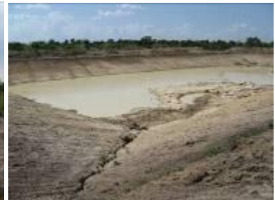
Olelpec dam under construction, Apac
