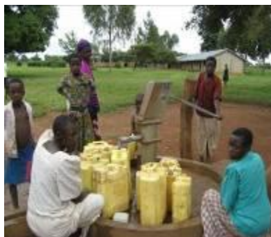
Rehabilitated borehole in use, Wamulongo Primary School, Mayuge
