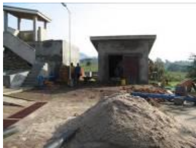
Remaining works underway prior to commissioning of the PWSS, Kamwenge
