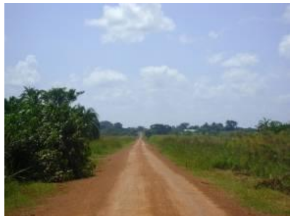
Picture shows swamp filled using force account on Masindi – Rwenkunya road
