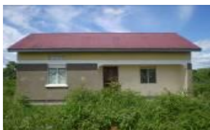
Completed staff house at Kungu HCII
