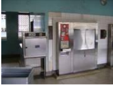
Renovated sterilization unit
