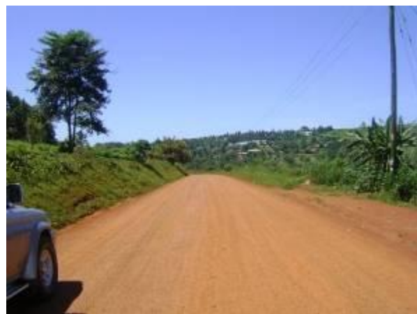
Picture shows a completed section done by force account on Lugazi – Buikwe road
