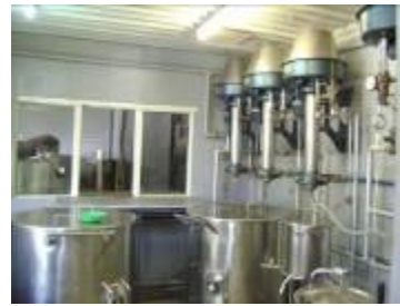
Renovated intravenous fluids plant
