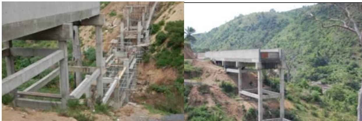
Construction of aqueducts at Mpanga HEP dam
