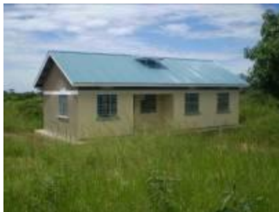
Staff house at Muhembiro HCII
