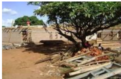
Medical ward under construction
