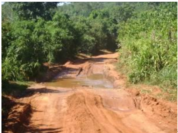
Picture shows a section of Lubugumu – Bugigi road in Mukono district where periodic maintenance was done
