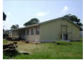
Laboratory under renovation
