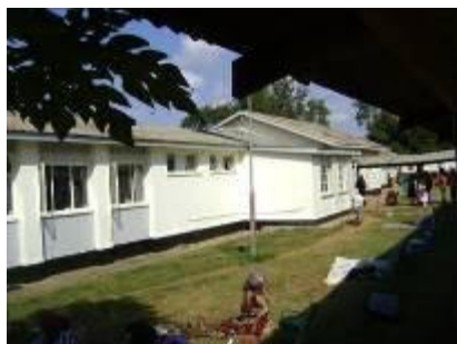
Rehabilitated maternity ward
