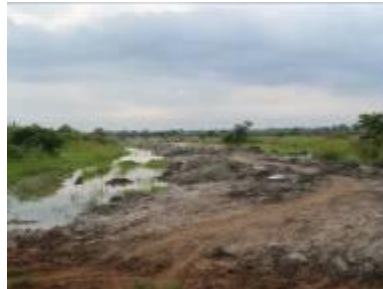
Impassable road leading to Olamia valley tank, which needs to be rectified by the contractor, Apac
