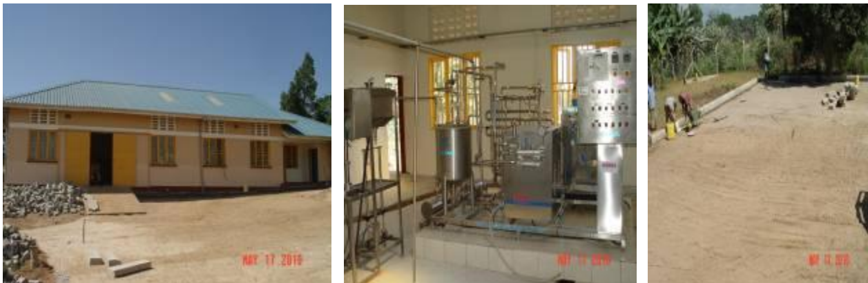
Front view of Nabusanke Fruit Factory plant, installed equipment and ongoing paving
