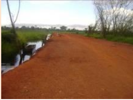
Works in progress: Swamp filling across Mpongo River
