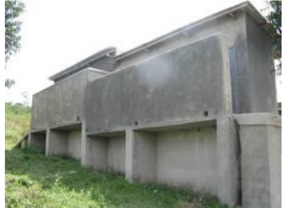
Construction of an ECOSAN facility at Kimuli Secondary School, Rakai district
