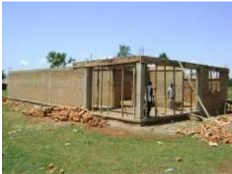
Construction of the drug store
