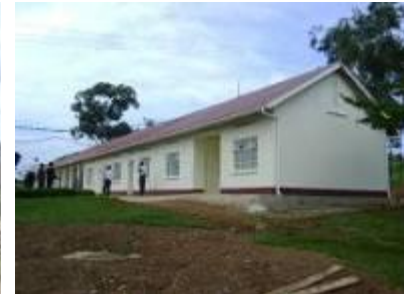
Renovated and expanded admin department
