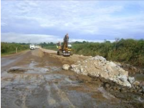
Busega – Masaka Road: Swamp widening (left) and Dust control by routine watering (right)
