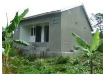
Staff house at Namungo HCIII
