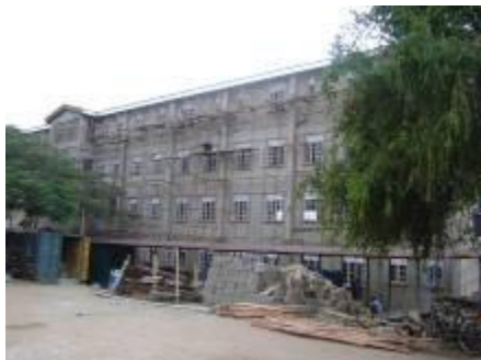
3 storey medical ward
