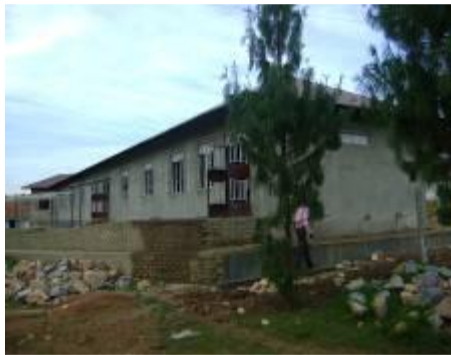
Male TB ward under renovation&
