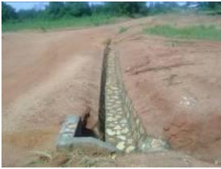
A stone lined drain along Nakazi – President's lodge road
