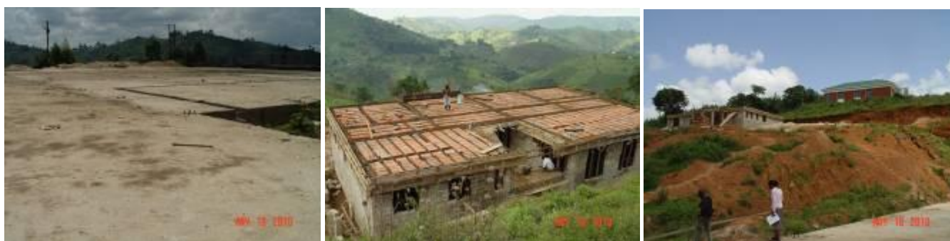
Main plant slab, administration block and kitchen house at Burere-Buhweju
