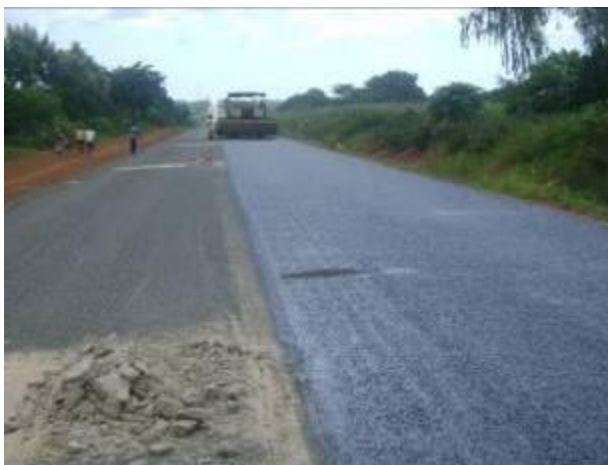
Dokolo – Lira road: Works in progress - 2 nd layer of bituminous surface dressing (left) and stone lining of open drains in Dokolo town (right)
