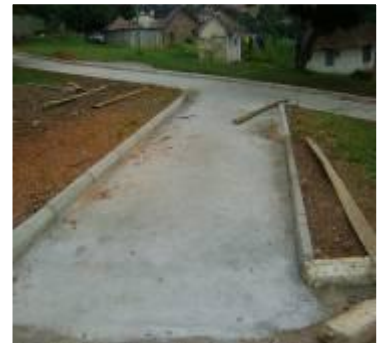
Paved access roads
