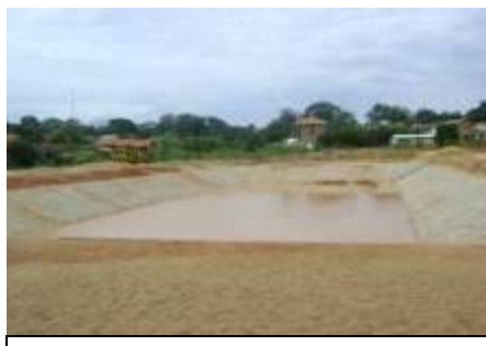
Lagoon under construction
