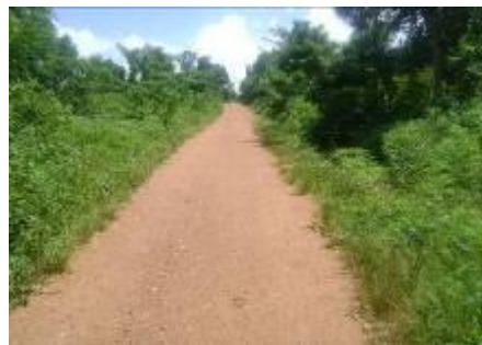
A completed section of Ddekabusa – Luwuube road with overgrown shoulders
