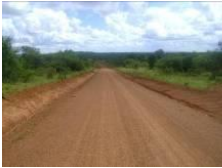
A completed section of Ntantamukye – Kaweema road
