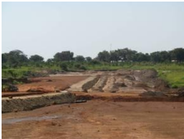
Works ongoing on Akwera dam, Otuke district
