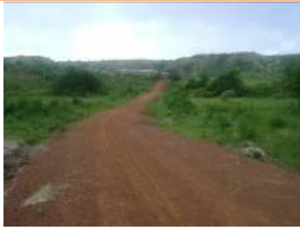
A completed section of Endiizi – Mpikye road
