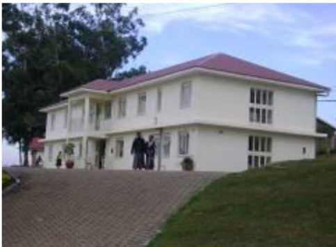
Completed private ward
