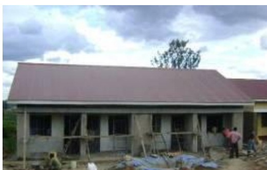
Staff house at Lwebitakuri HCIII
