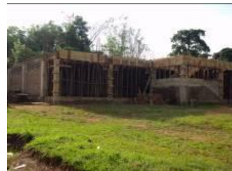
Storied classroom block
