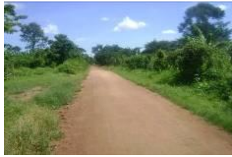
A completed section of Kigavu – Balida road
