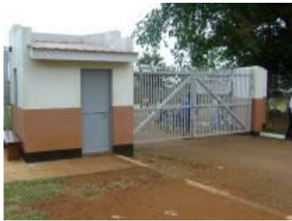
New gate and security house
