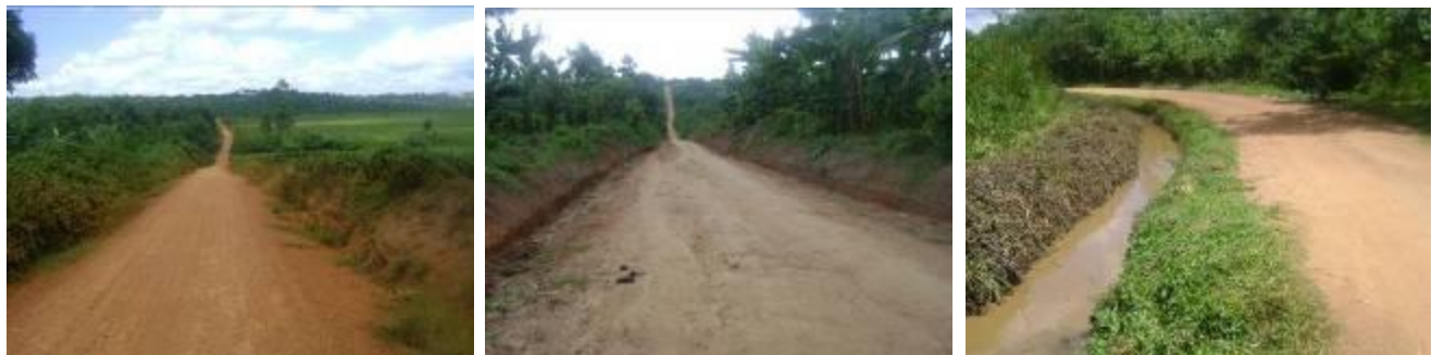
A completed section of Buswabulongo – Nama road, still in good condition (left); a bush cleared section of Nsozibiye – Kiwawu road under LGMSD (center); and a section of Wabiyinja – Nsozibiye road with a manually opened side drain (left).
