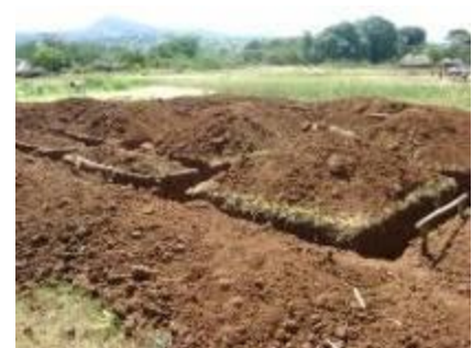
Staff house at Pagwata HCII
