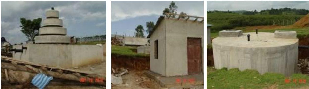
Water filter, pump house and water tank at the Irrigation plant
