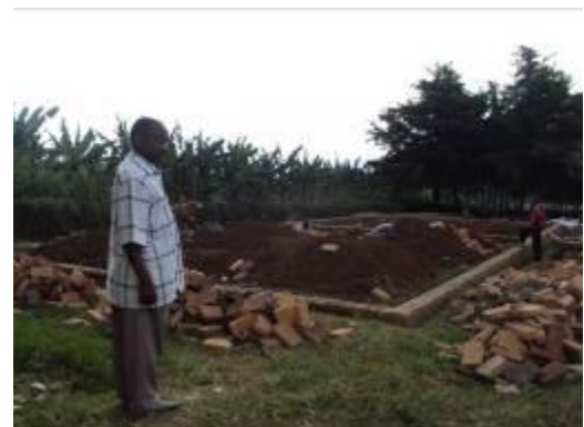
Science Lab. at substructure
