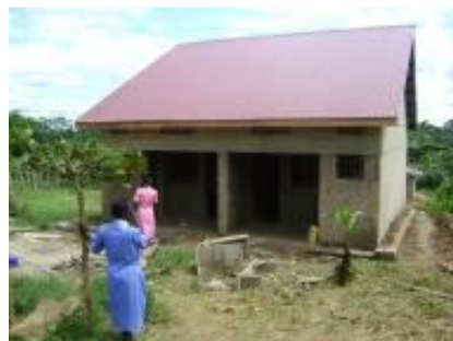
Staff house at Kalangalo HCII
