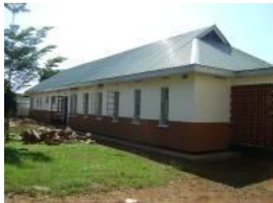
Male ward under rehabilitation
