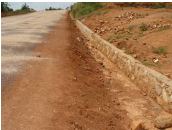
Incomplete By pass link, parked trucks (out of fuel), and primed Kyaliwajala road with stone pitched side drains below
