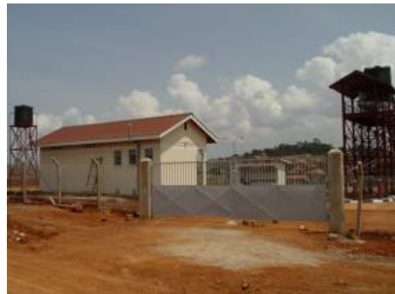
Completed calibration rig, fence and water system at Bweyogerere
