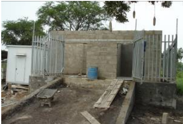
New Transmission Site under construction at Eregu
