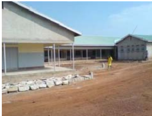
Jinja district PHC Development: completed phase II at Kagoma hospital (top left and right);
