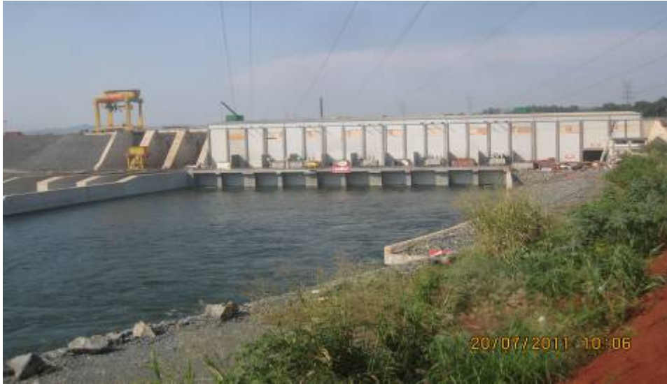
Overview down stream
