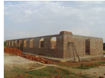
Dormitory block at ring-bim level
