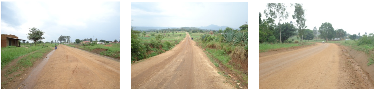
FIGURE 4 HEAVILY CORRUGATED SECTION AT 0+100 (KATRINI), COMPLETED GRADED SECTIONS OF THE ROAD AT 5+400 AND WIDE SECTION OF THE ROAD AT 19+500 ON THE APPROACH TO NYADRI
