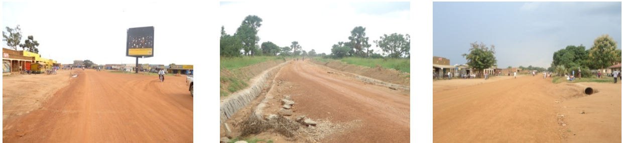
FIGURE 2 COMPLETED SECTION AT 0+000 (KOBOKO TOWN), STONE PITCHED DRAINS AT 7+400 AND INCOMPLETE ACCESS CULVERT INSTALLATION AT 28+300 (KURU TC)
