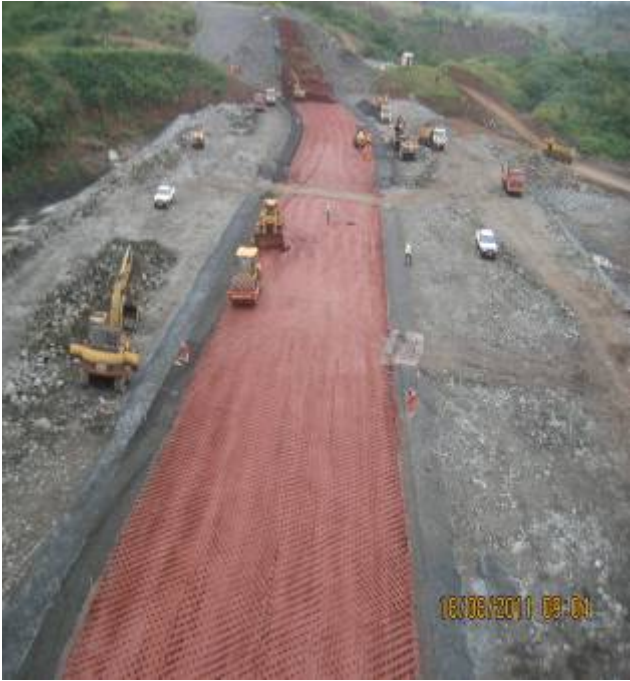
Earthworks, right Embankment
