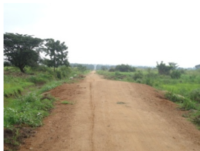
FIGURE 5 ROAD OPENNED UP AT NAGONGERA (0+000) AND SWAMP CROSSING AT 3+600 LIKELY TO IMPEDE TRAFFIC IF DRAINAGE STRUCTURES ARE NOT PROPERLY INSTALLED AND SWAMP FILLED TO OVERCOME FLOOD SITUATIONS.
