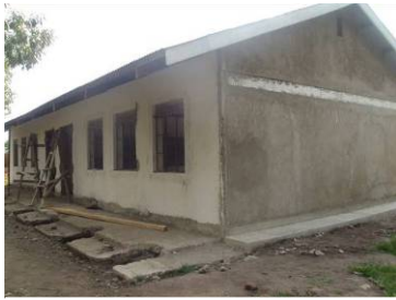
Classroom block under completion
