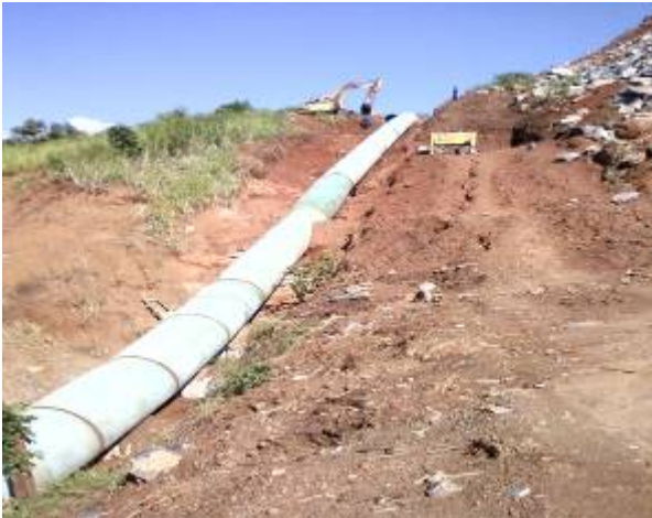
Nyagak HEP: ongoing works on the Penstock;
