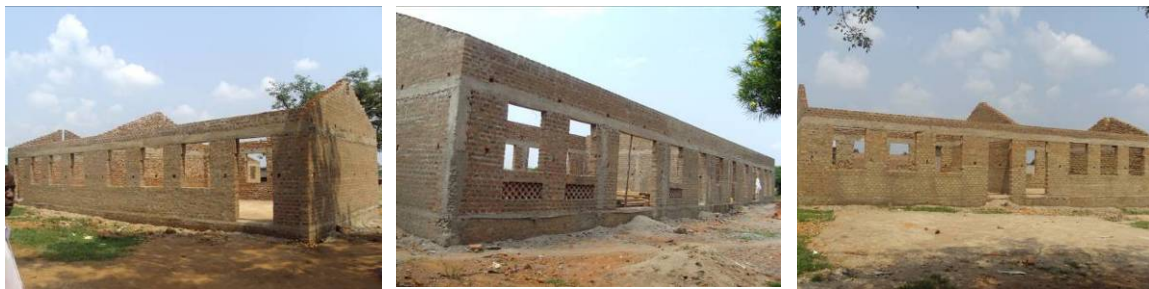
A 2 classroom block, a CJ and BCP workshop and another 2 classroom block at roofing level.
