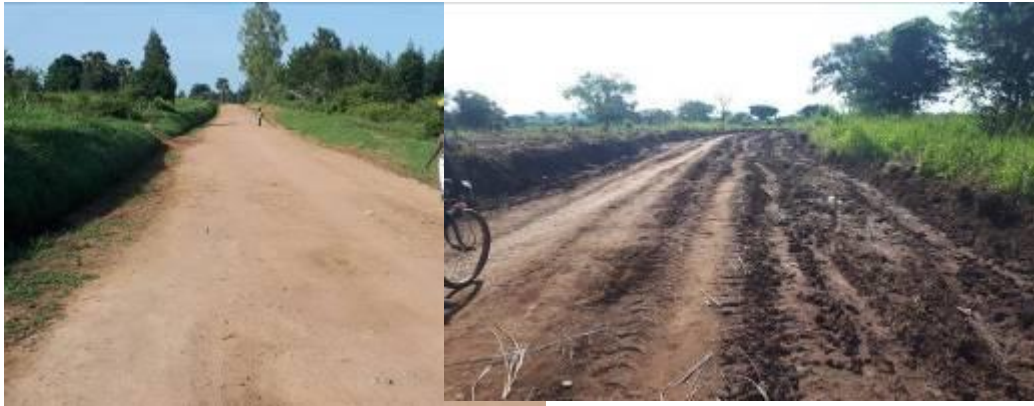
Eruba-Logiri Road (23km) after grading and gravelling works in Q4 FY2017/18
