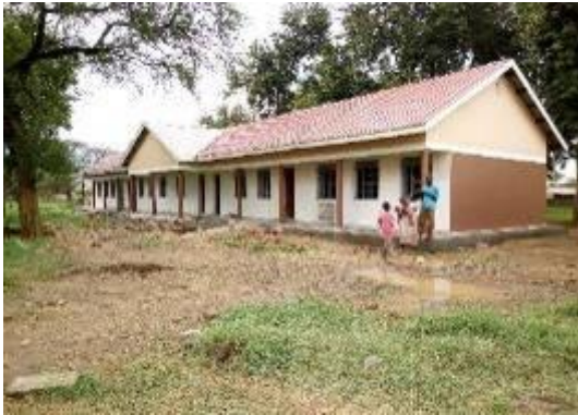
Functional Classroom Block at Lorengedwat Primary School in Nakapiripit District
