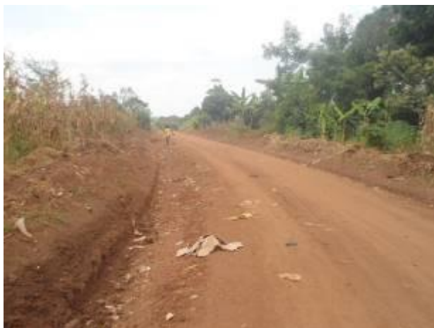
A graded and shaped section of Kakoni-Mpigi-Nakafumu road
