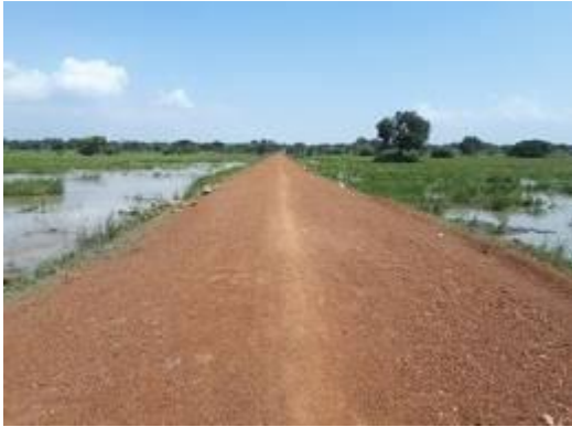
A raised swamp section along Soroti-Omugenya –Odela-Obule Road (7.4 km)
