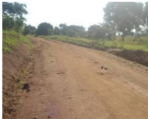
A graded and shaped ssection of Mabuye-Nakakono road with loose material
