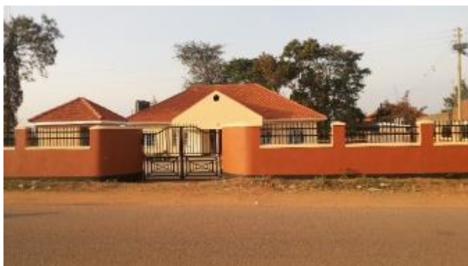
Non-functional Support to Luwero- Rwenzori Regional Office at Luwero district headquarters
