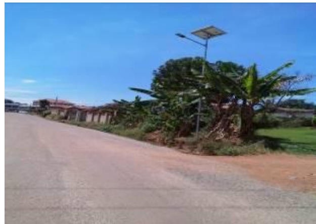
A section of Kiwafu close showing the paved surface and one of the installed street lights
