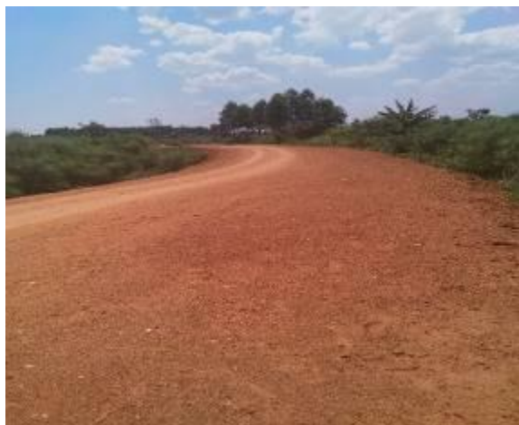
A filled section of the Kabuhuna swamp crossing
