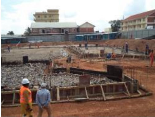
On-going formworks at Soroti Market site
