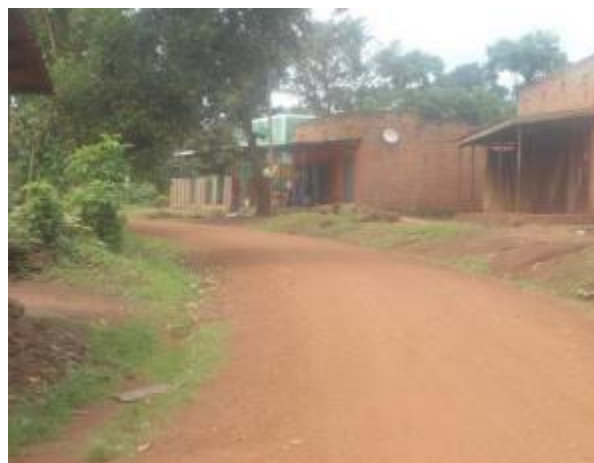
A section of Family Spirit - Kamurasi road at km 0+000
