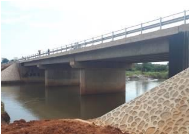
Pager bridge across river Pager along Kitgum – Musingo road
