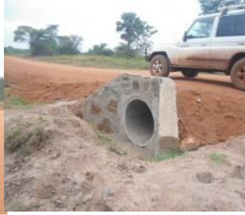
An installed culvert with end structured on Ihungu-Bulyamusenyu road at km 39+500
