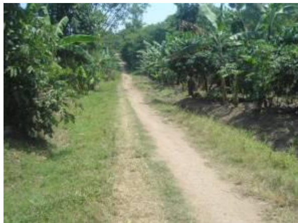
A section of Ruyenda-Kitooma-Rumuri that required routine manual maintenance works
