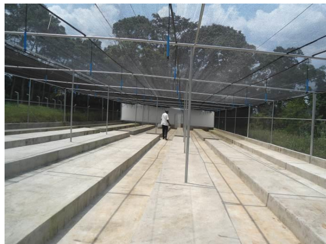
Completed screen house ready for use at NaCORI, Mukono District
