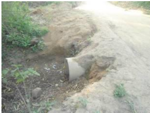
A culvert installed along Lwentama-Kisoma-Mijunwa road at km 0+100
