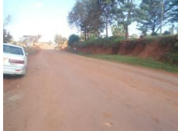
A graded and shaped section of Busabala – Kaazi Road at km 1+600
