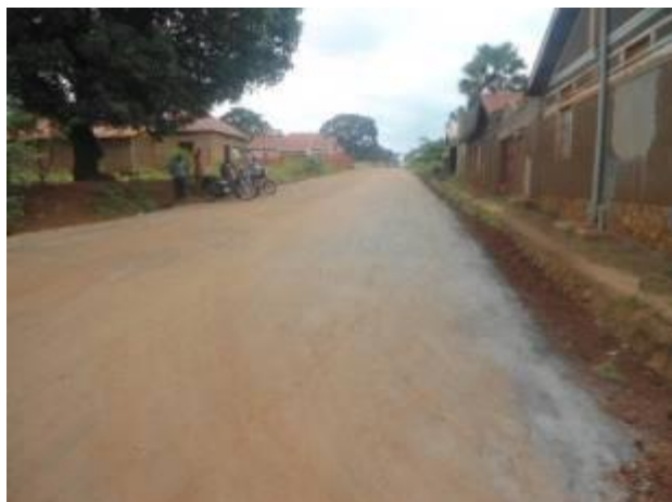
A primed section of the Hospital Road
