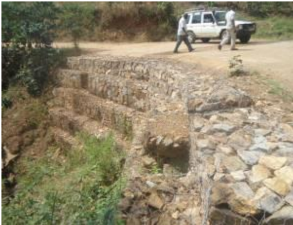
Gabion Embankment works along Ruhumuro-Burungira-Kikorijo-Nyeibingo-Buhimba road
