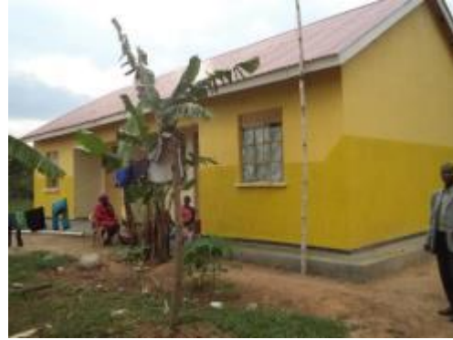
New residence of the teacher's house in Serere district
