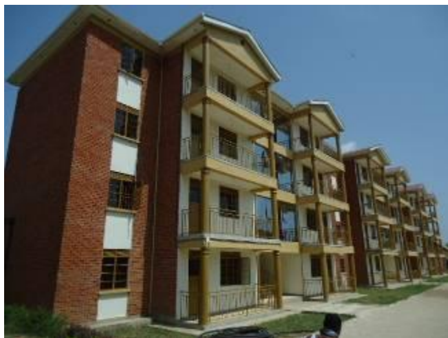
Completed staff houses at Soroti RRH
