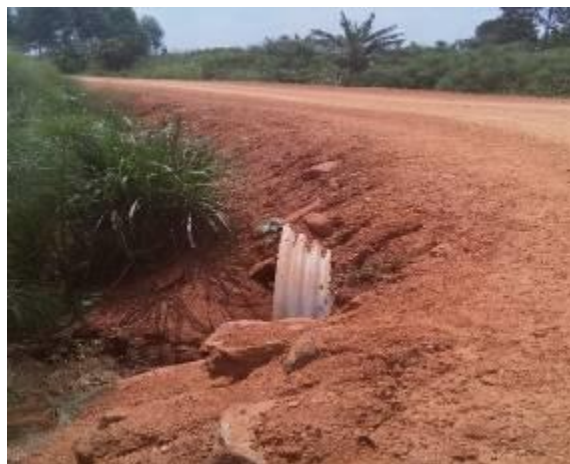
An installed armco culvert along the filled section
