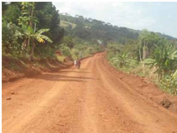
A section of Luyannzi-Kasubi at km 4+000
