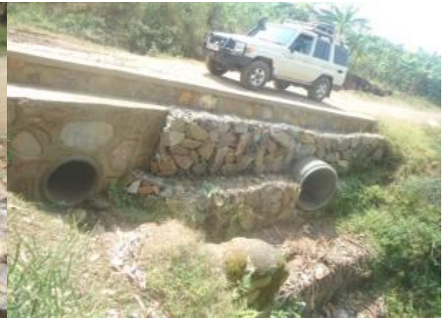
A double line at km 3+600 along Nyaruzinga-Bumbaire-Kitabi (10.km)
