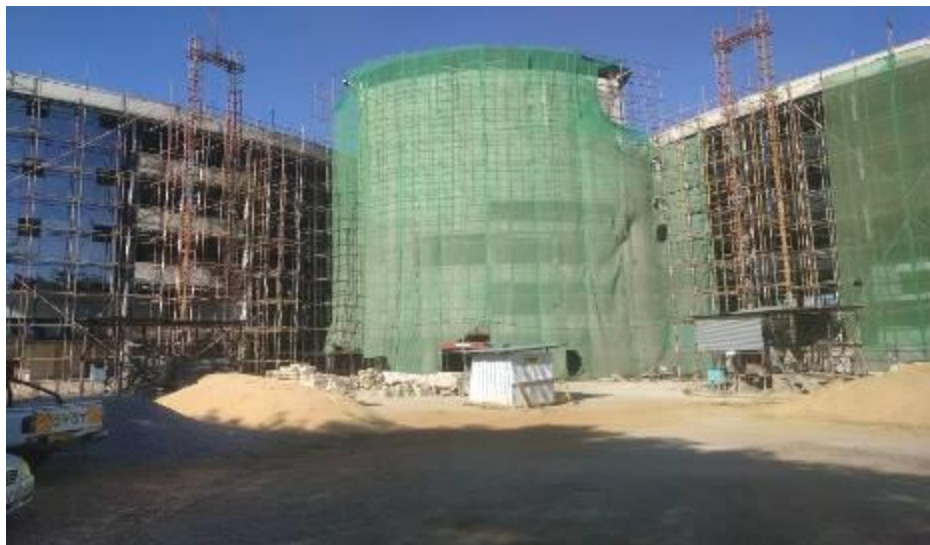
Ongoing finishing works for phase 3 for the Petroleum Directorate building
