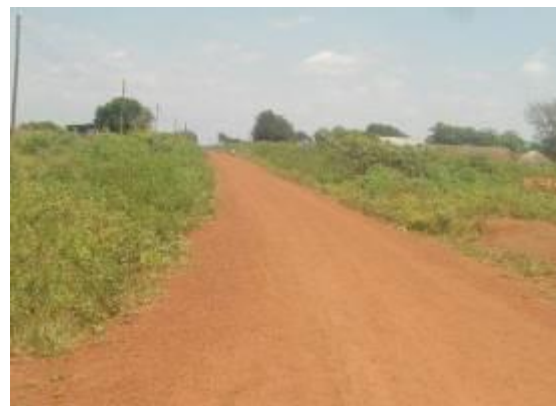
A well rehabilitated section of Jeja-Kinyara road at km 3+400
