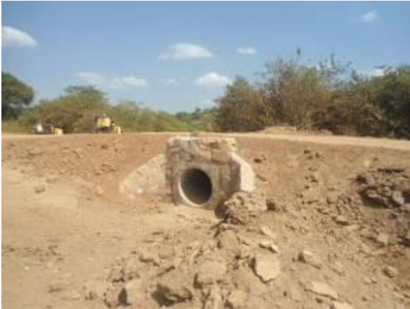
A culvert at km 10+700 on Kasambya-Nabakazi road
