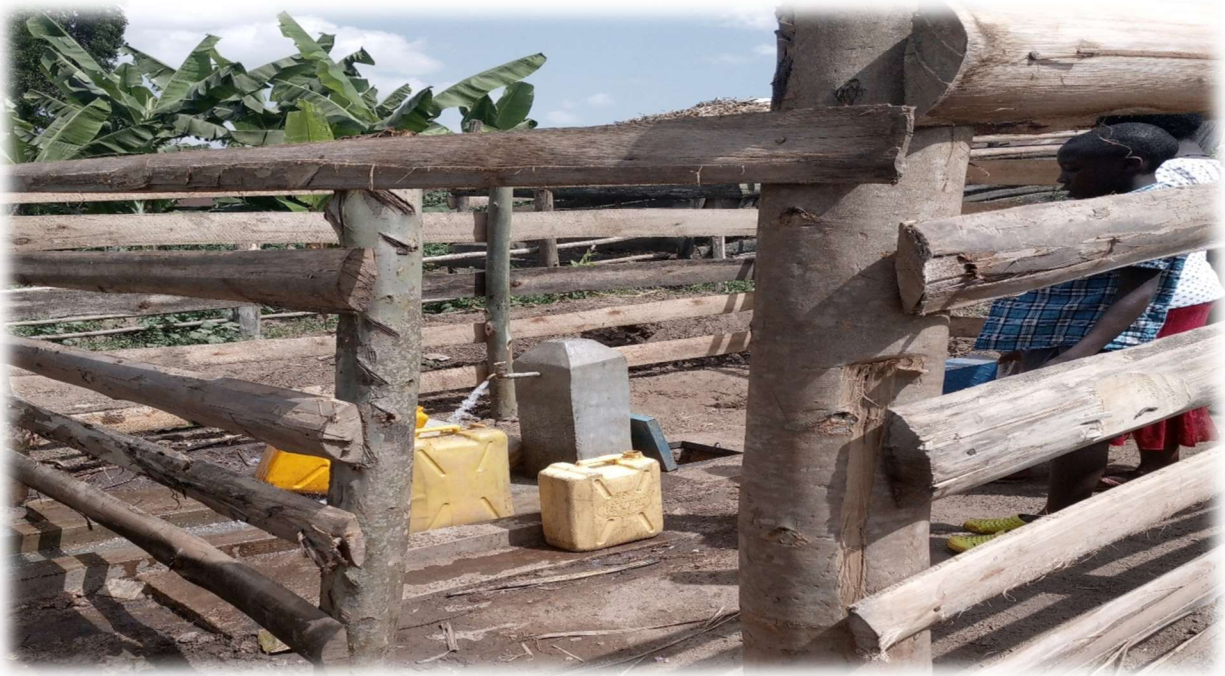
A single tap stand constructed near Birago's home on Kachwamuhoro pipeline.
