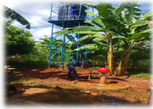
Installation of irrigation equipment in Bugiri DLG
