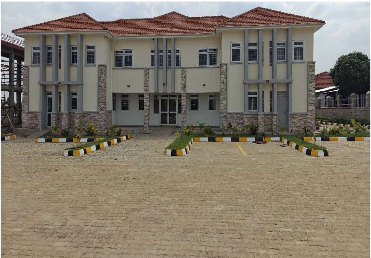
Photo Showing Progress on Construction at Hoima Blood Bank – Front View
