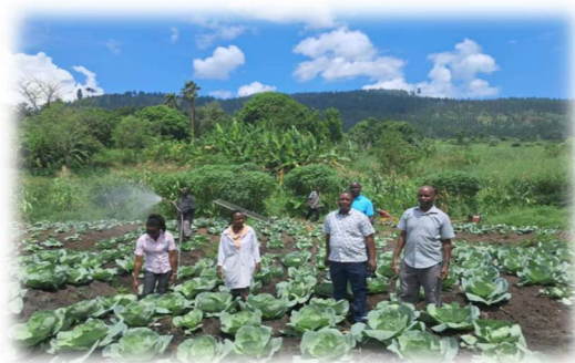
Solar powered irrigation system installed in Jinja
