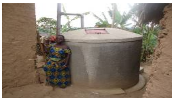
L-R: Ongoing construction of Ferro cement tank by Katosi Women; A Ferro cement tank constructed by Shuuku Development Cooperation
