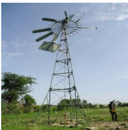
L-R: Non-functional windmill for pumping water and tap stand at Rengen in Rengen Sub-County
