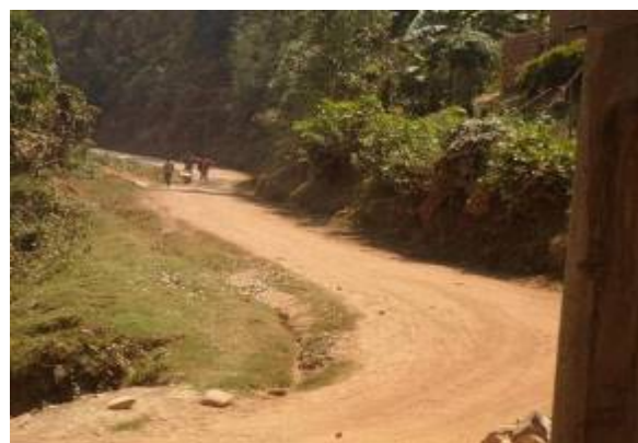
Graded section along Katuna–Muko road maintained by force account
