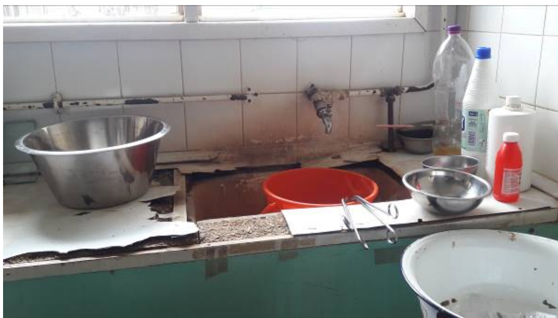
A sink at Pallisa General Hospital
