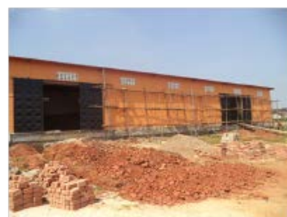
Outside works at Namanve stores
