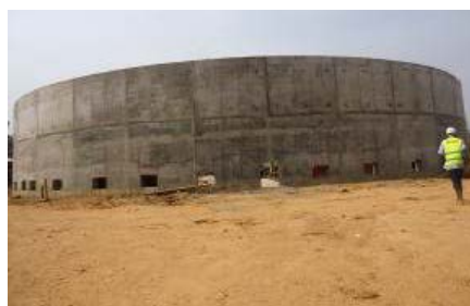
A Trickling filter at Bugolobi, Kampala
