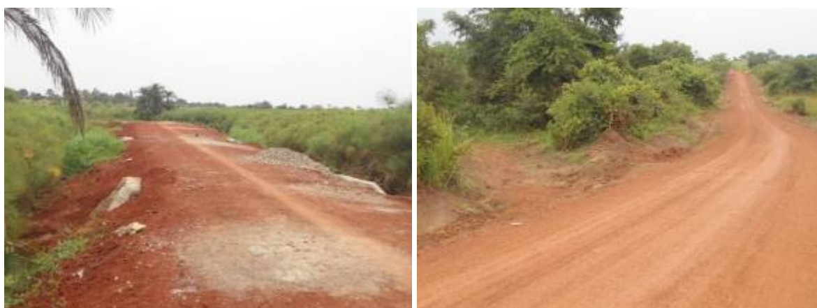
Left: A raised swamp section at Km 4+100 along Koro-Rom-Pece road; Right: A gravelled section with an off shoot drain along Palenga-Willacic (18km) road which was due for hand over
