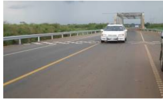
Part of the completed and handed over Kalagi–Mukono section at Sezibwa river along Mukono–Kayunga road
