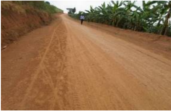
A gravelled section of the Mabona-Kicuzi-Rwabatenga road
