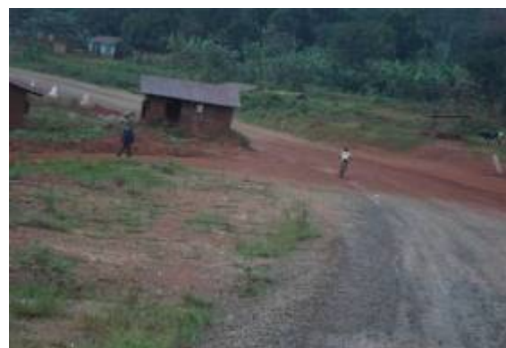
Semi-permanent house within the ROW where owner has denied contractor access on the Mpigi-Kanoni road
