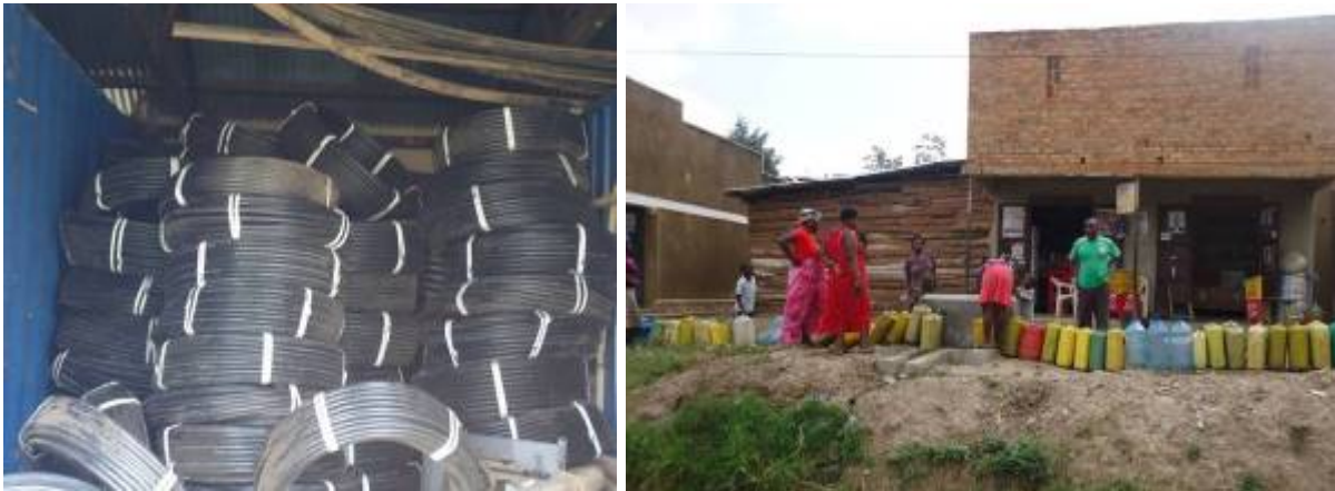
R: Some of the pipes delivered for the extension of Makanga WSS in Kabale district; People fetching water at a PSP in Ruti-Rugando WSS. Mbarara district
