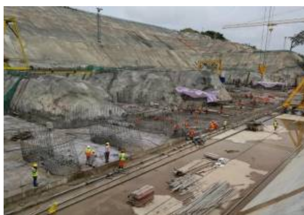
Civil works at the power intake
