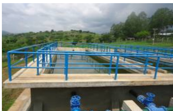
L-R: Section of sedimentation tanks of Nyarwodho GFS; A water jar constructed by Busoga Trust
