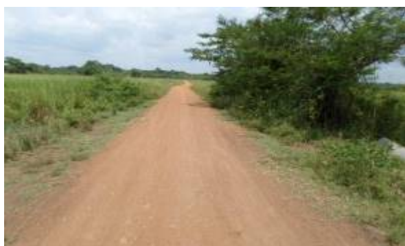
A completed section along Namunkanga–Nabutaka road
