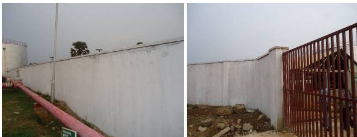
Wall fence constructed at Jinja storage tanks in awaiting final finishes
