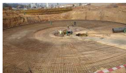
Base steel works for one of the secondary sedimentation tanks in Bugolobi, Kampala
