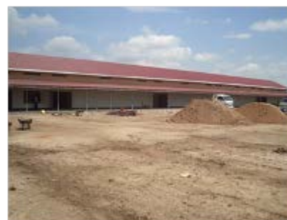
Left: Completed stores in Namalu Prisons, Nakapiripit District
