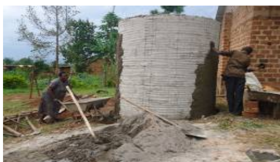
L-R: Ongoing construction of Ferro cement tank by Katosi Women; A Ferro cement tank constructed by Shuuku Development Cooperation
