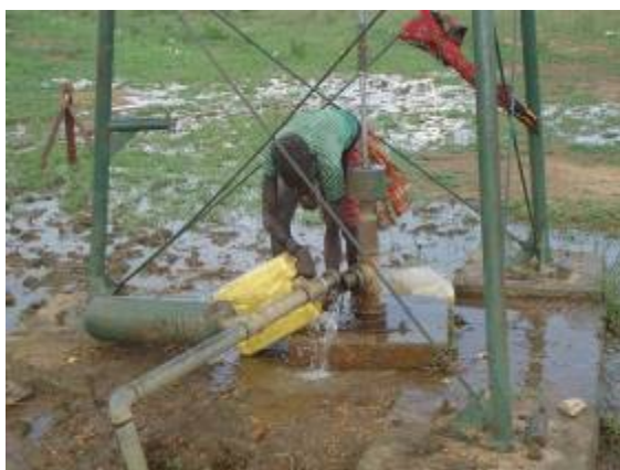
L-R: Energy service provider at his store with Energy saving stoves; Leaking Pipes at the partially restored windmill for pumping water in Lokitalebeu Sub County in Kotido district
