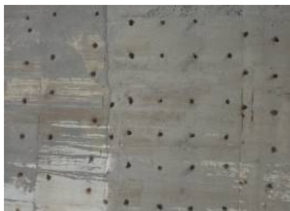
L-R: Contractor removing non recommended formwork ties; Holes created upon removal of the formwork ties before being filled at Isimba HPP
