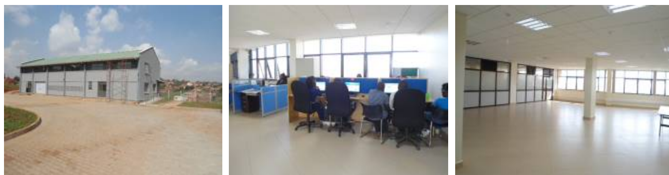
Completed warehouse, furnished 2 nd floor and the 4 th floor of UNBS headquarters
