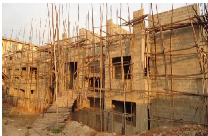
Staff quarter construction under construction at Mbarara RRH
