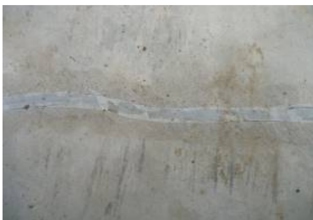
L-R: Repaired crack at the stilling basin of the spillway; Civil works at the Embarkment Dam at Isimba HPP
