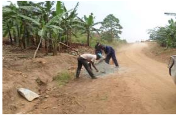
Preparatory works for construction of the culvert end structures
