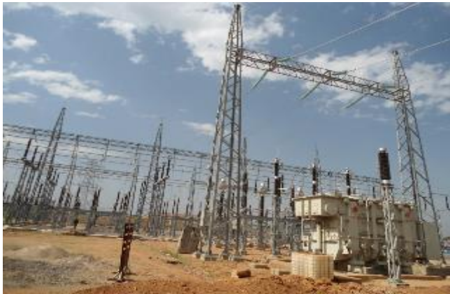
L-R: On-going equipment erection at the 132/220kV New Mbararara substation; On-going civil and electro-mechanical works at Mirama Hills substation
