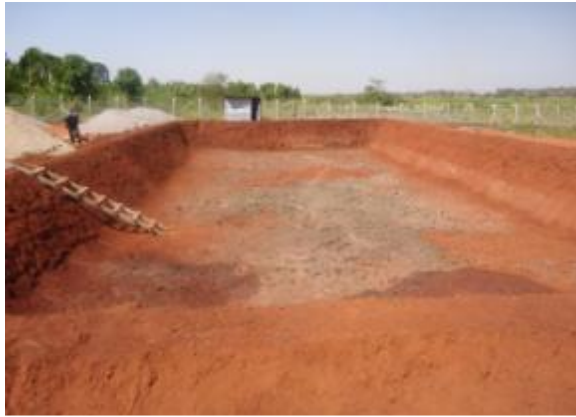
L-R: Excavation for the Sludge Drying Bed; Anaerobic Baffled Reactor tank of Kayunga Faecal sludge in Kayunga district
