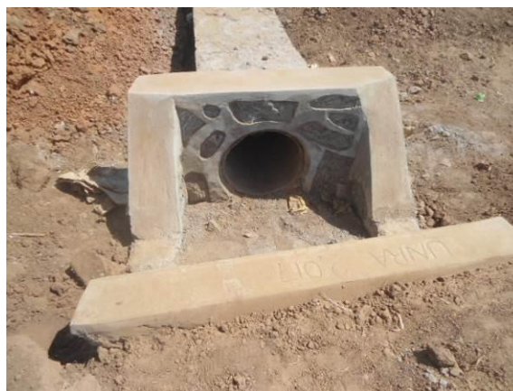
Installed culvert pending backfilling along Aduku-Nambieso Road
