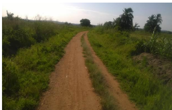
Bush covering part Bulingo-Kalangala landing site road due to lack of routine manual maintenance
