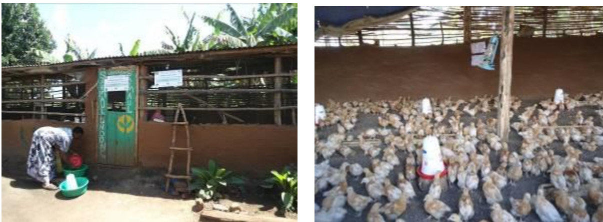
Poultry house constructed and stocked with chicks using the Saemaul Undong Korean model in Kiwumu A village, Kamengo sub-county, Mpigi district
