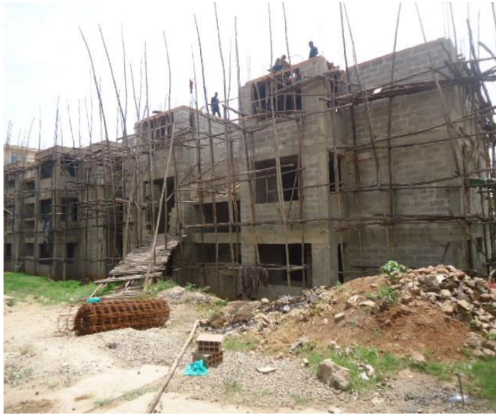
On-going construction works for staff houses at Mbarara RRH
