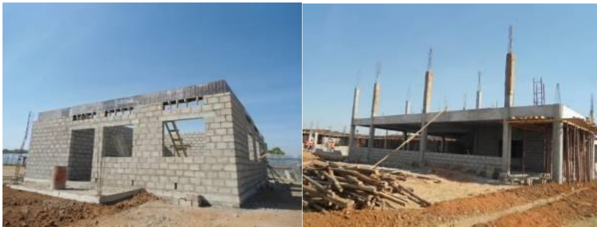
L-R: The Utility Block at 60% progress; and Science Block at 50% progress at Muni University
