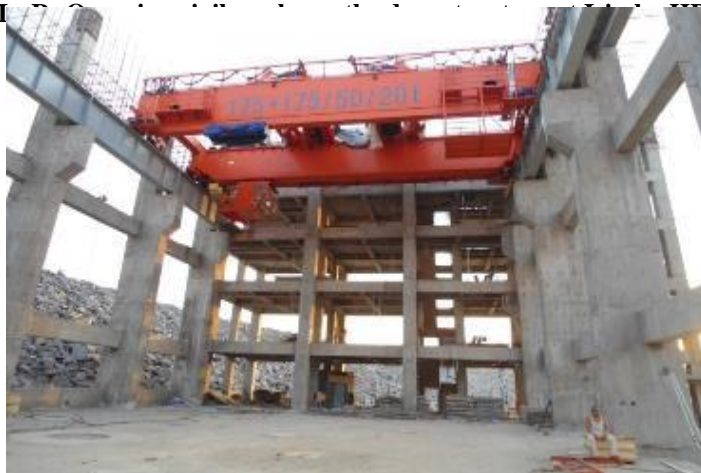
L-R: Newly installed Over Head Electric Crane in the machine assembly room; Repaired crack on part of the dam tailrace structure at Isimba HPP
