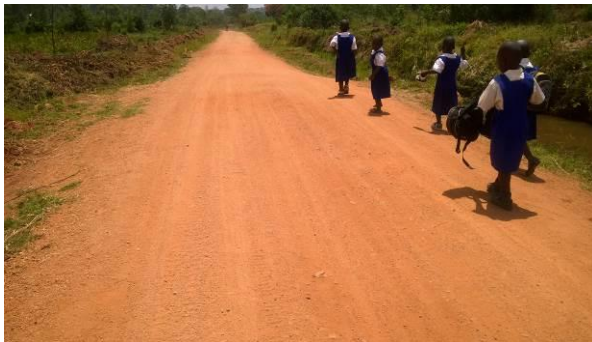
Graded section along Kalule-Bowa-Nakaseke – Kiwoko Road
