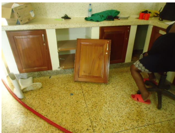
Left: Poor quality terrazzo and misfitted cabinet doors in the theatre at Nakaseke GH; Right: Poorly fitted theatre light at Atiak HC IV, Amuru District
