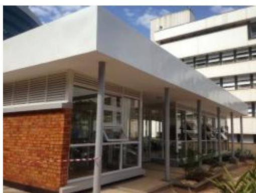
Left: Constructed client care shade at KCCA main offices in Kampala
