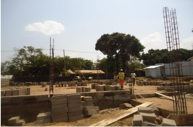
On-going construction works for the drug store at Arua RRH
