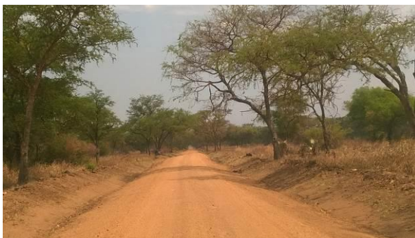
A gravelled section along Karugutu – Ntoroko road within the Murchson Fall National Park
