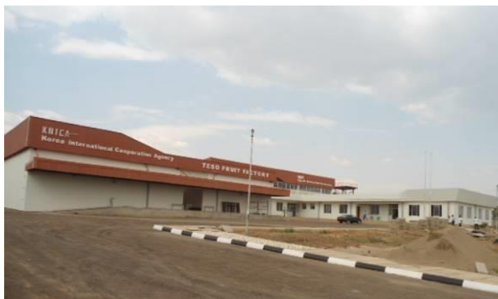
Completed civil works at the Soroti Fruit Factory in Arapai, Soroti district
