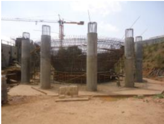
L-R: Reinforcement bars and columns of the Sludge digester; Scrapper bridge fitted in the primary sedimentation tank at the NWWTP in Bugolobi, Kampala district
