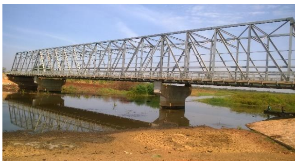
Finished deck for Kabaale bridge, Kyankwanzi district
