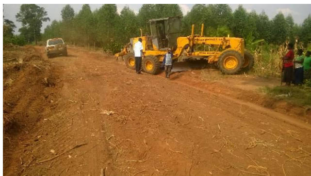
Grading works ongoing along RusandaraRwensambya-Muntabu-Kitoma
