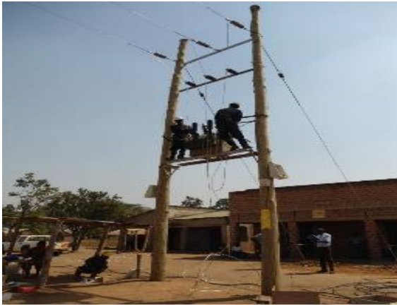
L-R: Workers of C&G Installing a transformer at Acuta Trading Center (Oyam District), Completed work on the Aduku-Inomo 33kV distribution line in Apac District
