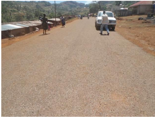
Completed second seal works on Moi Road in Kapchorwa Town Council
