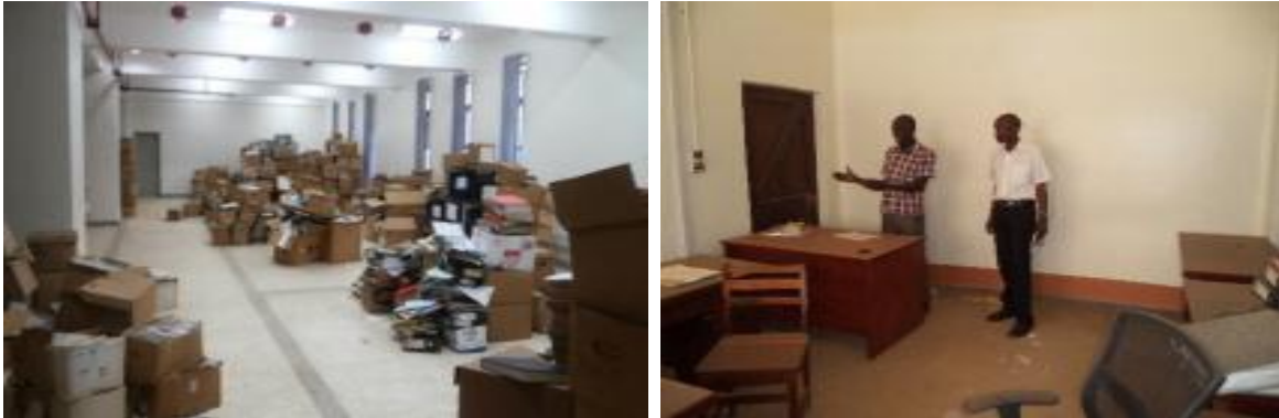
Left: Boxes of records on floor due to inadequate mobile shelves at the NARC building; Right: Vandalized IPPS centre in Soroti district
