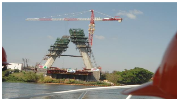
Construction of Pylon 2 of the New Nile Bridge in Njeru town
