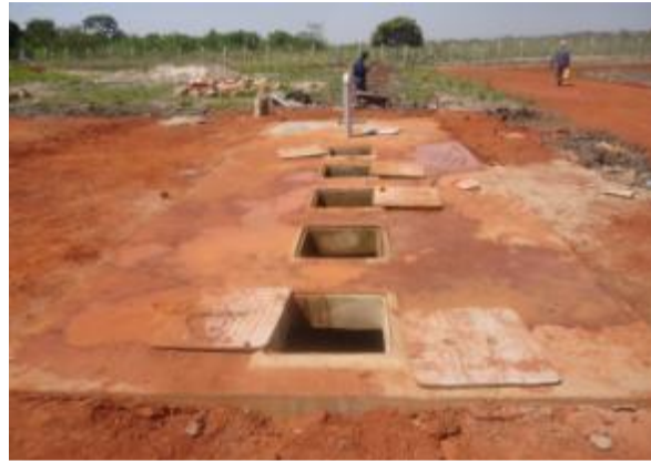
L-R: Excavation for the Sludge Drying Bed; Anaerobic Baffled Reactor tank of Kayunga Faecal sludge in Kayunga district
