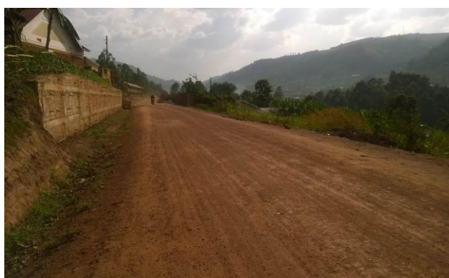
Stabilised gravel base for Bukinda-Highland tarmac road awaiting surfacing
