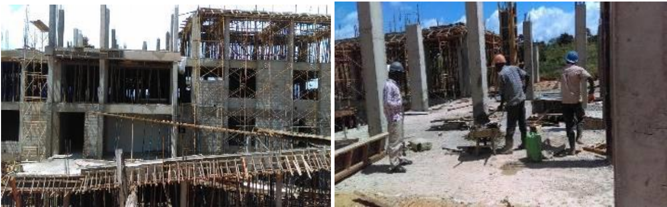
L-R: Construction works of new Engineering Workshop at ring beam level with structural works completed at 90% at Kyambogo University
