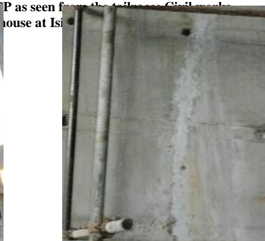
L-R: Newly installed Over Head Electric Crane in the machine assembly room; Repaired crack on part of the dam tailrace structure at Isimba HPP
