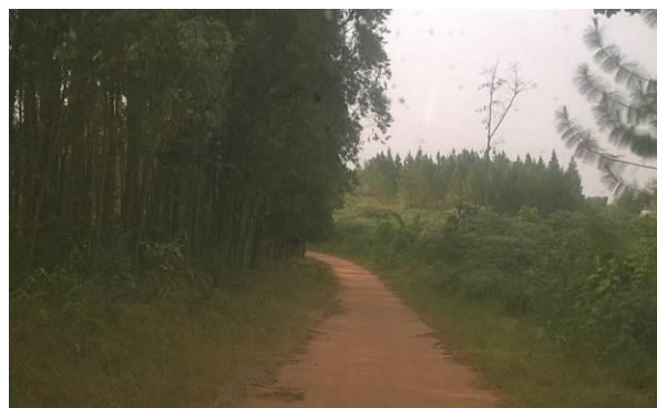
Kyakatwanga-Kakwaku-Kisenge road under routine manual maintenance
