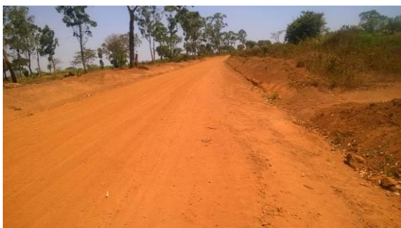
A gravelled section of Ihungu-Bulyamusenyu Road (42km)
