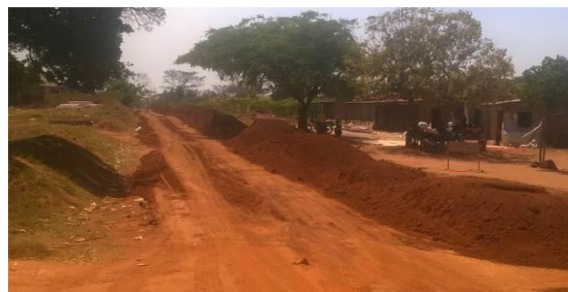
Gravelling works on going along Ikooba- Ntoma Road
