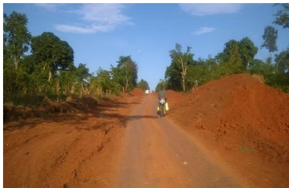
Bush clearing along Bukulula–Kalungu Road – a pilot project for full gravelling
