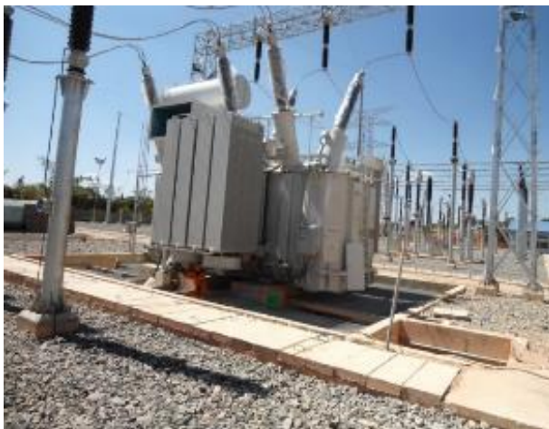
L-R: Installed 250MVA transformer at the 220kV section; Ongoing external works on the partially completed 220kV plant house at Kawanda sub-station
