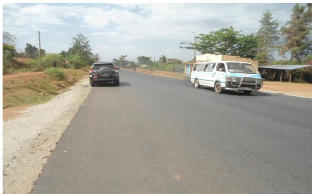
A trial asphalt section along Namunsi-Kapchorwa Road
