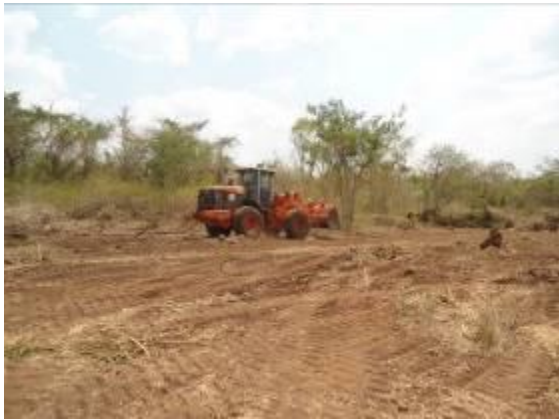
Bush clearing was ongoing at AMFRI FARM in Nakaseke district
