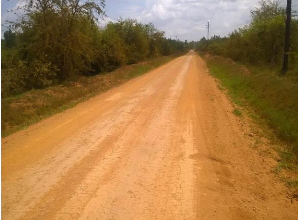
Gravelled section for the term maintenance contract of Villa Maria–Kyamulibwa – Kabulasoke Road
