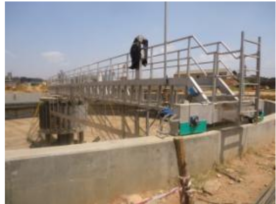
L-R: Reinforcement bars and columns of the Sludge digester; Scrapper bridge fitted in the primary sedimentation tank at the NWWTP in Bugolobi, Kampala district
