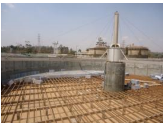
L-R: Laying of filter material in the trickling filter; A section of the grit removal chamber at the NWWTP in Bugolobi, Kampala district
