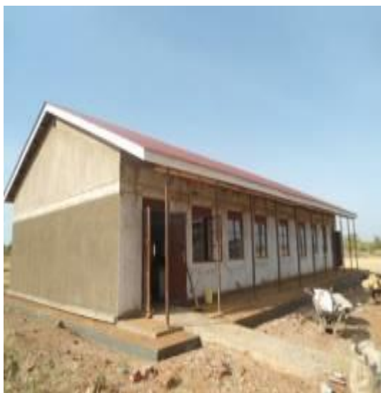
A science block completed at Patong S.S in Agago district
