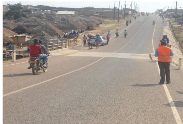
A completed section of Ali-Keny Road in Koboko town
