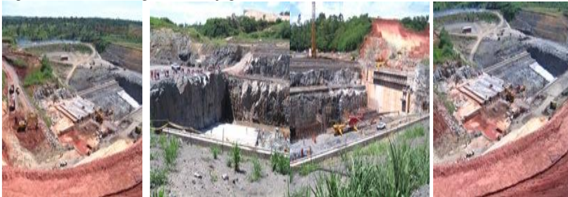
Figure :Works in Progress on Bujagali Dam Wall Construction October 2008
