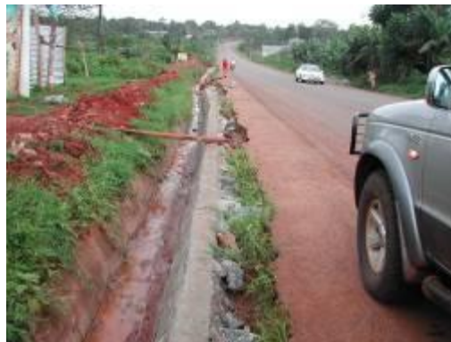
Photos show on going quarry works and erosion of the shoulders due to laxity in protecting completed works
