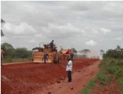
Photos show ongoing works during the site visit: Mechanical stabilization of the sub-base
