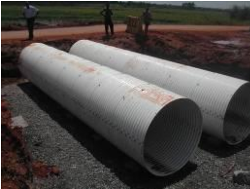
Photos show culvert installation and GCS base construction works in progress during the site visit
