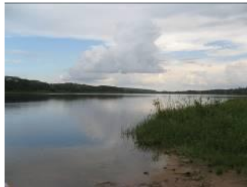
Kakinga dam completed
