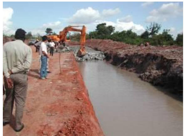
works in progress during the site visit: extension of existing culverts and rock-fills in swamps
