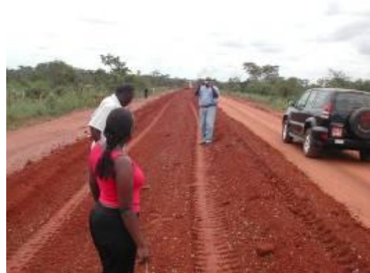
Photos show ongoing works during the site visit: Mechanical stabilization of the sub-base
