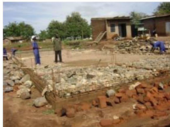
Market buildings at Rhino Camp, first half at ring beam and second half at hardcore and blinding level
