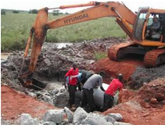
works in progress during the site visit: extension of existing culverts and rock-fills in swamps
