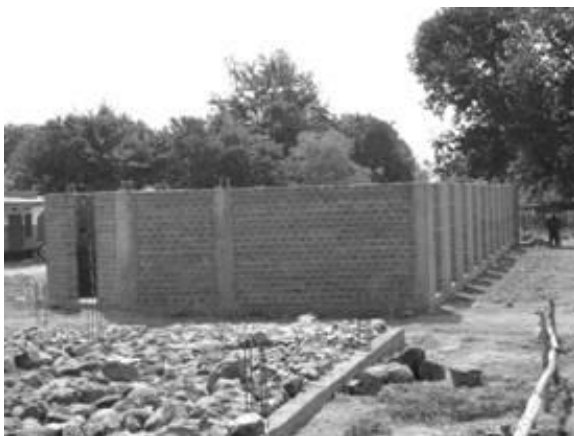
Market buildings at Rhino Camp, first half at ring beam and second half at hardcore and blinding level
