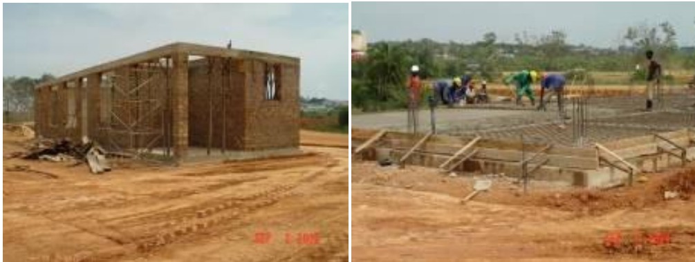
Engineers' office and construction of the floor slab for KIBP offices-Namanve
