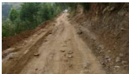
Grading in progress along the road
