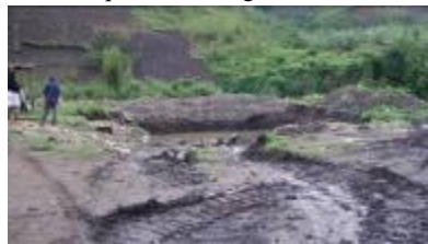
Excavations for the foundation of the bridge.
