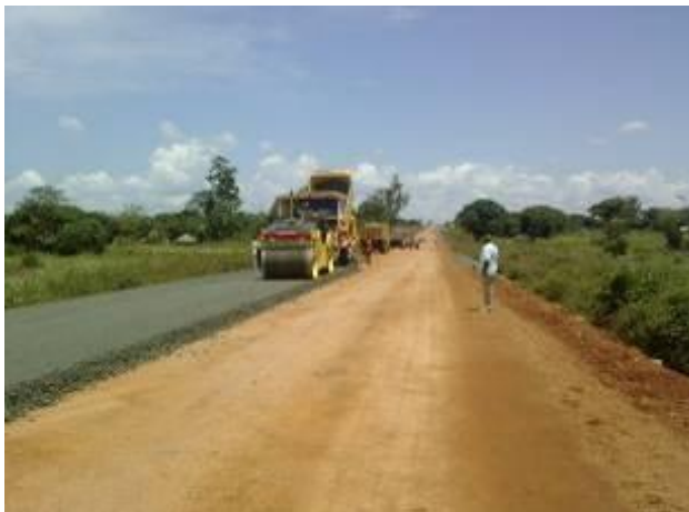
Soroti – Dokolo road: Placing of the last 500m of base layer (Left) and a section of the primed surface (right)
