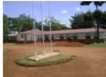
OPD remodeled into Administrative Building
