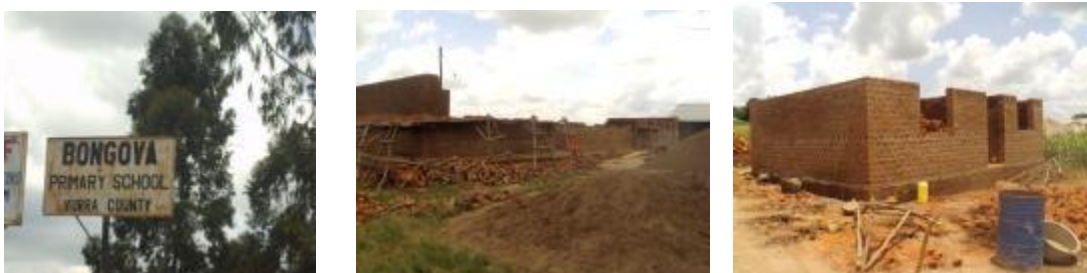
A 3 classroom block and a teacher's under construction
