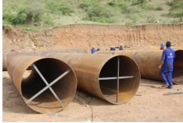
Construction works at Forebay and Penstock pipes at Buseruka HEP.
