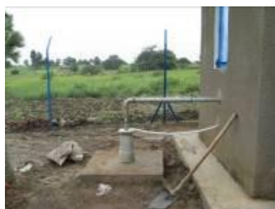
Production well for the piped water system, previously used as a community borehole, Koboko piped
