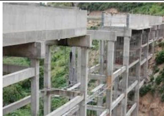
Construction works on Dam/Weir and channel on aqueduct at Mpanga HEP.
