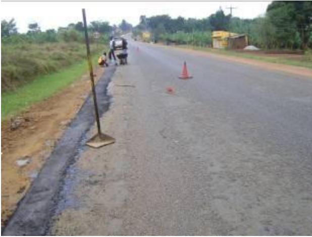
Masaka – Kyotera Road: Edge repair with a bitumen slurry seal
