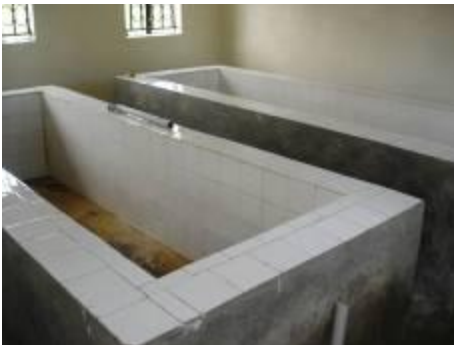
Completed hatchery in Koboko
