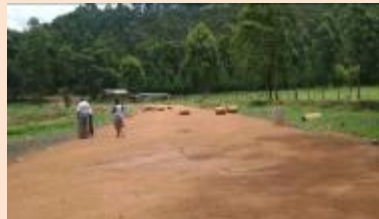
Gravel fill allowed time to settle
