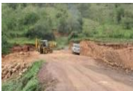
Evidence of works ongoing, at Kagango dam, Isingiro district
