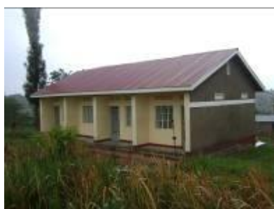
Staff house at Lwengo HCIV
