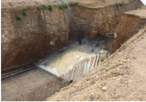
Construction works at Forebay and Penstock pipes at Buseruka HEP.
