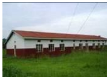
Maternity ward not in use
