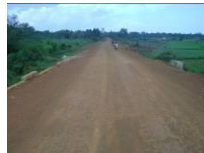
Namayingo – Nankoma road: completed section done by contract
