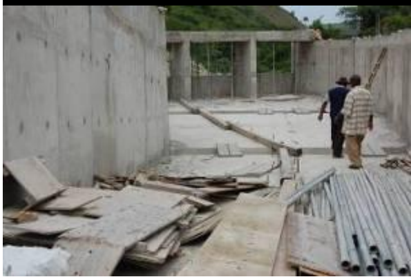
Channel (intake) on Mpanga HEP dam
