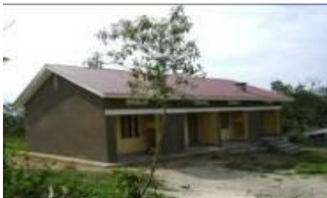
Staff house at Kibalinga HCIV
