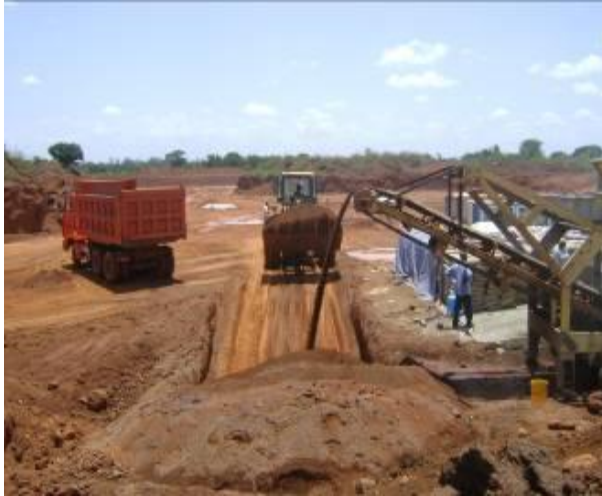
Dokolo – Lira road: Mixing of gravel with cement for the Sub-base layer (Left) and a section of the compacted sub-base (right)
