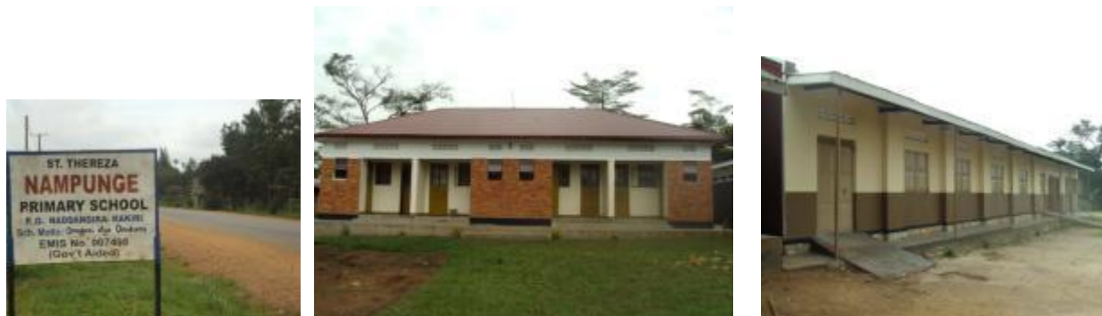
A staff house and a classroom block that was completed at Nampungwe P/S
