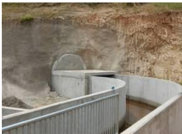
Channel entrance into the tunnel
