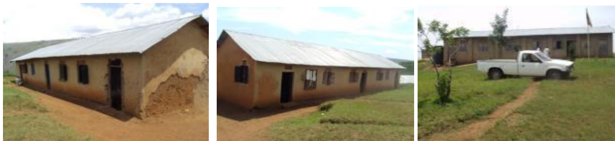
The structures on the land at Karungu S.S. procured at Ushs 326,910,000/=
