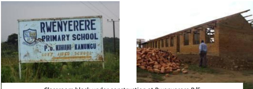
Classroom block under construction at Rwenyerere P/S
