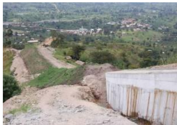
Aerial view of Penstock and Powerhouse
