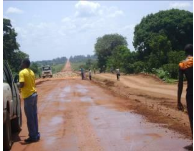
Dokolo – Lira road: Mixing of gravel with cement for the Sub-base layer (Left) and a section of the compacted sub-base (right)
