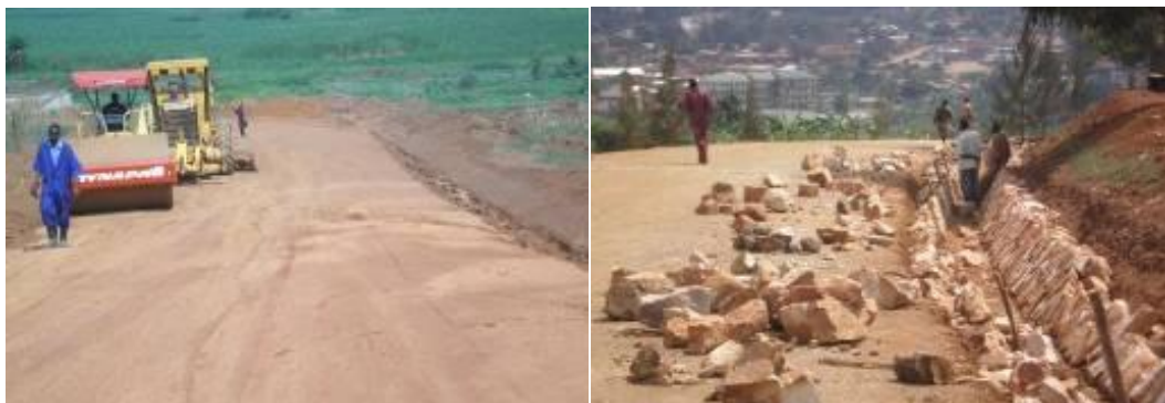
Graveled section of the road and drainage works at Luzira
