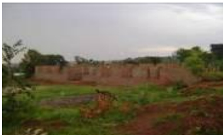
Maternity ward at Kaserem HCIII
