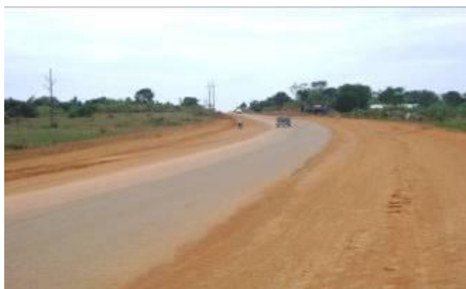
Busega – Masaka Road: Section widened for a climbing lane (left) and earthworks for widening of swamp areas (right)
