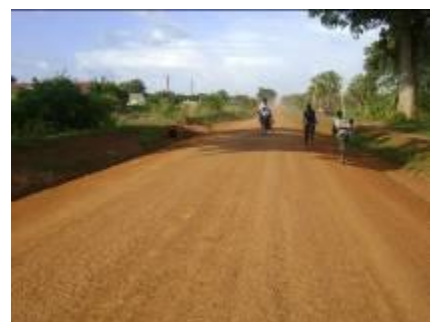
Soroti – Serere road: completed section of the road
