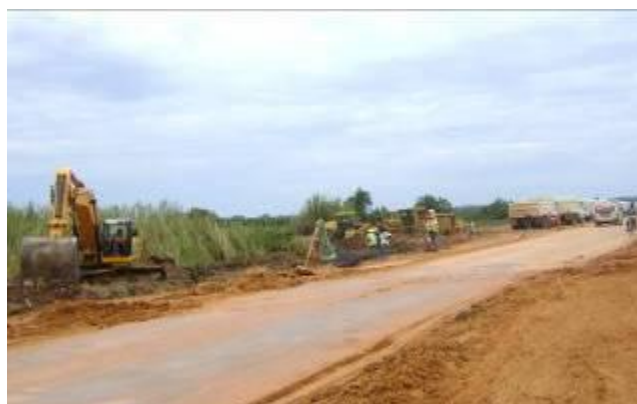
Busega – Masaka Road: Section widened for a climbing lane (left) and earthworks for widening of swamp areas (right)
