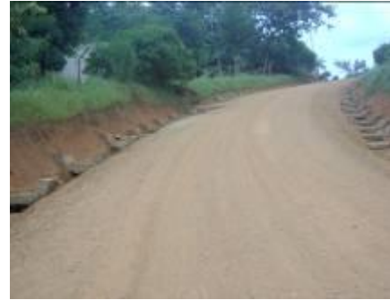
Namagumba – Budadiri: Section of the completed road
