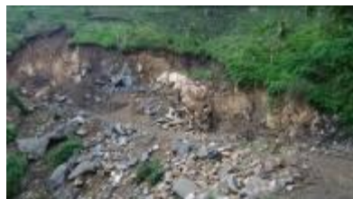
Section of access road to the bridge, which required blasting
