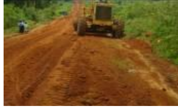
Gravelling in progress
