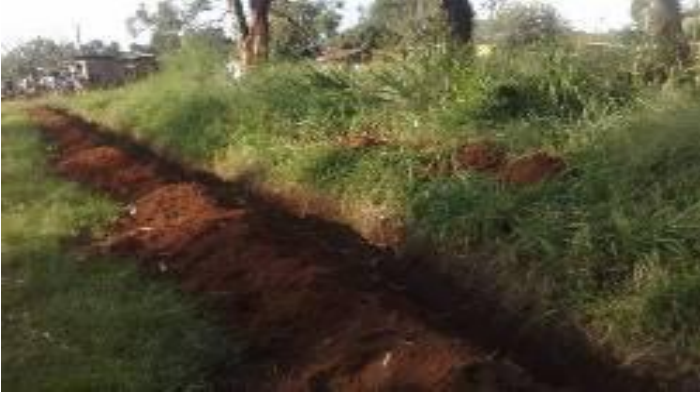
Evidence of pipe laying in Minakulu Subcounty, Oyam district
