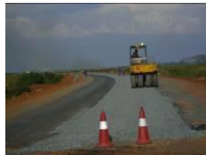
Soroti – Kumi road: Surfacing of the last 600m of Awaja swamp
