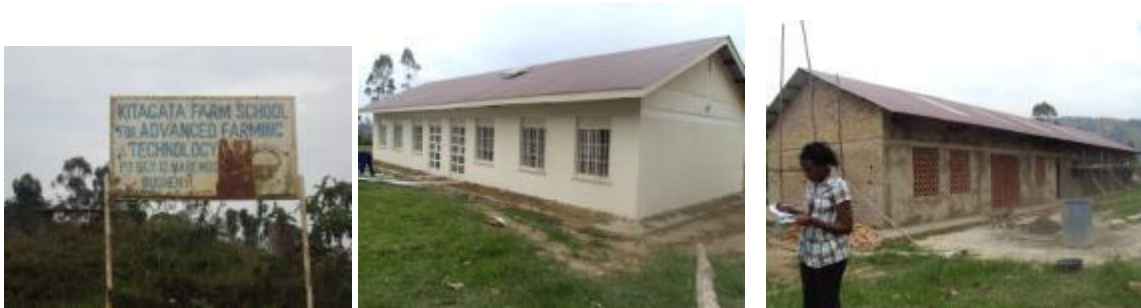
A completed classroom block and BCP & C J workshop at Kitagata
