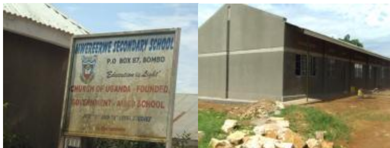
A 3-classroom block completed at Mwererwe S.S
