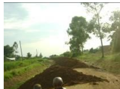
Magodes – Railway station road: on-going works done by Force Account
