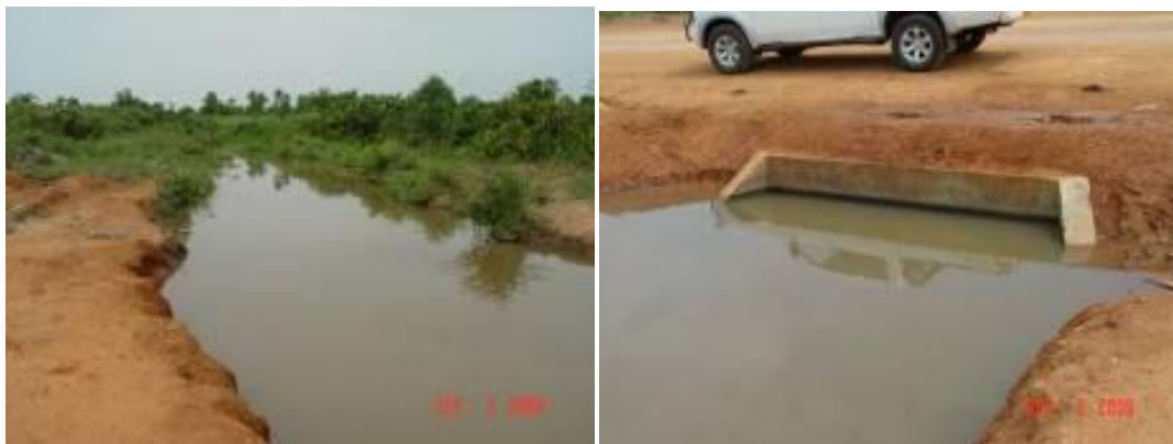
Blocked downstream of Namanve River causing backlog washing
