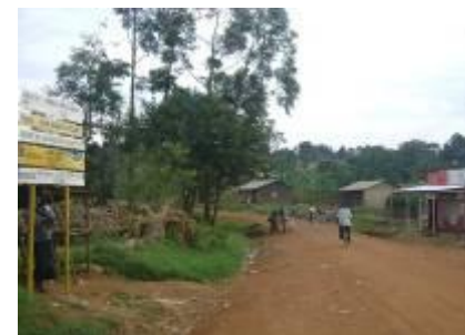
Nabumali – Busolwe road: A completed section done by contract
