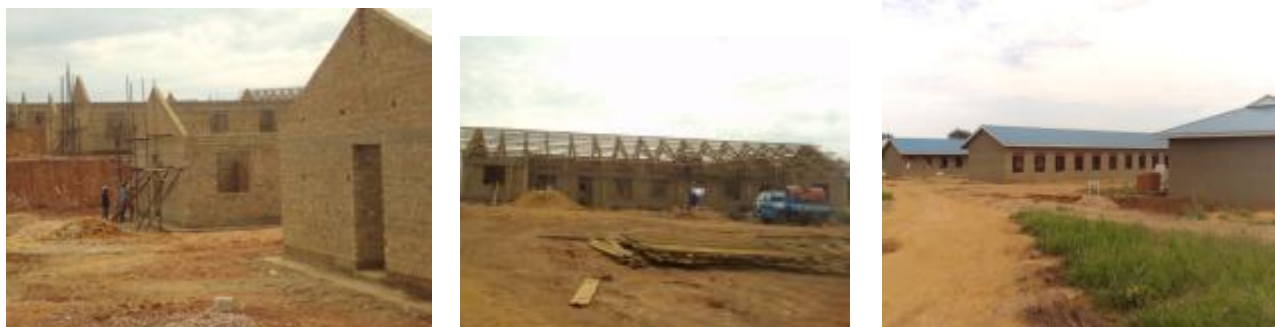
Dormitories, multipurpose hall and classrooms at Shimoni PTC
