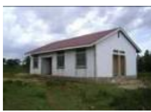
Staff house at Kanyumu HCII
