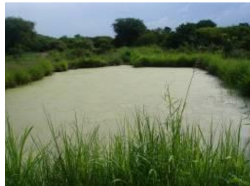
Suru Valley Dam in Arua
