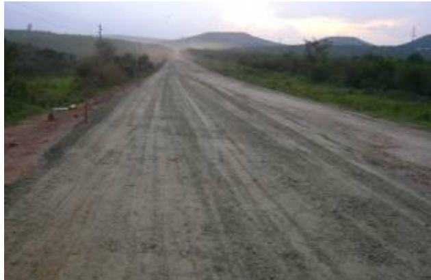
Masaka – Mbarara road: Section with a dense bitumen macadam layer (Left) and a section of graded crushed stone base (right)
