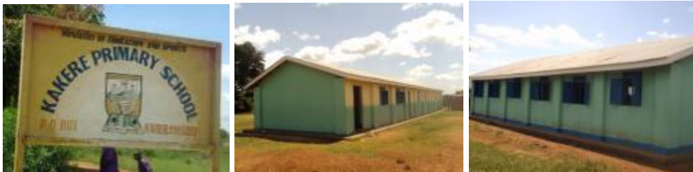
The classroom block that were walled at Kakere P/S at 45m
