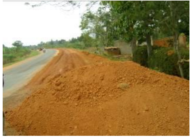
Nyendo – Villa Maria Road: Shoulder repair with a borrowed gravel material
