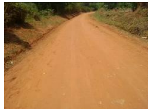
Kalule – Bamunanika: A section of the road recently graded using force account
