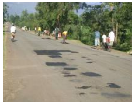
Namunsi – Sironko road: ongoing pothole patching with asphalt
