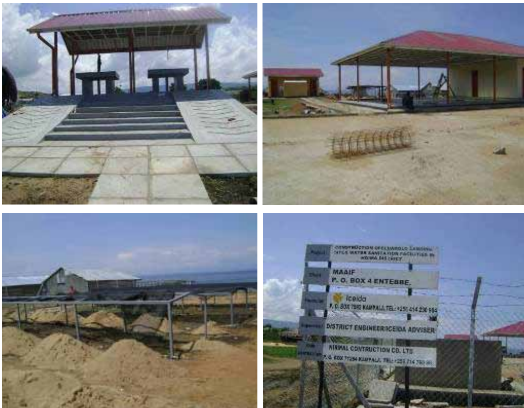
Civil works near completion at Sebagolo fish handling facility Hoima district
