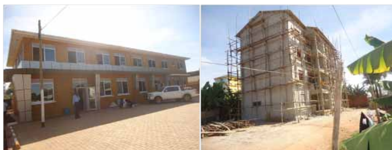
Left to right: Nearly completed administration block and staff quarters under construction Gulu RR hospital
