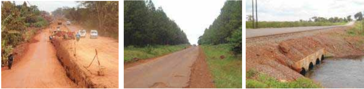
(Left); Embankment filling near Namulesa TC at Km 4+500. (Centre): A section of the road at Km 15+000 where works have not yet started. (Right); A completed section at a swamp crossing at Km 37+800.
