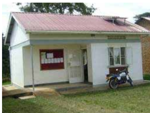
New DFO office block in Nebbi district
