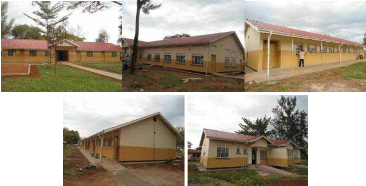
From the top left corner an administration block, a 501 seater main hall, a library block, a 3 unit science laboratory and a semi detached house all at completed at Bukedi College Kachonga.
