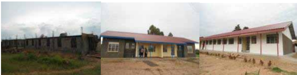
A storied dormitory block, the semi detached 2 bedroom house and the ICT laboratory
