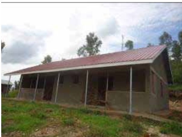
Left OPD construction at Iterero HCII Ntungamo district
