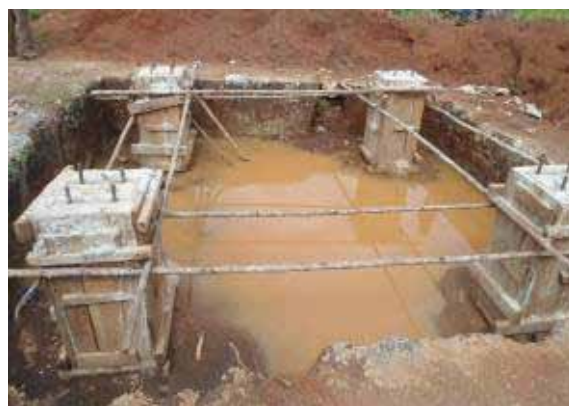
Tank basement for erection construction works
