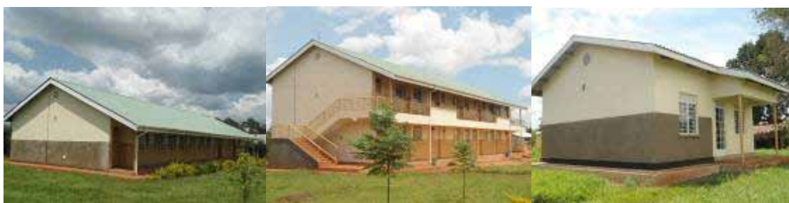
A library/computer laboratory completed, a storied 6 classroom block completed and 2 bed room house completed at Bukanga S.S
