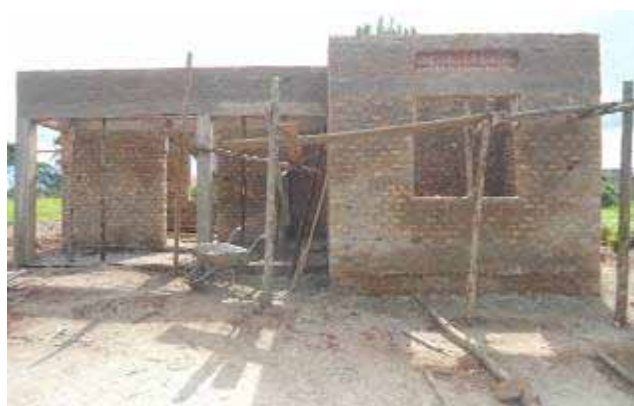
Kahunge Office block under construction
