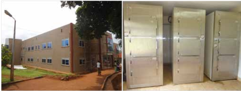
Left to right: Private wing under construction and repaired Mortuary fridges at Jinja RR Hospital
