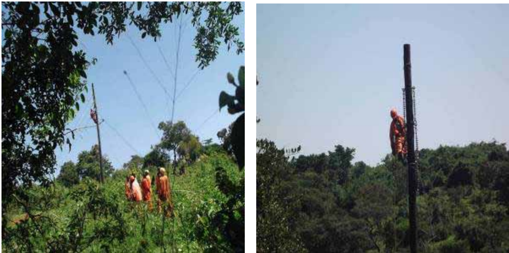
Stringing works ongoing on the Nkoge-Kashozi line
