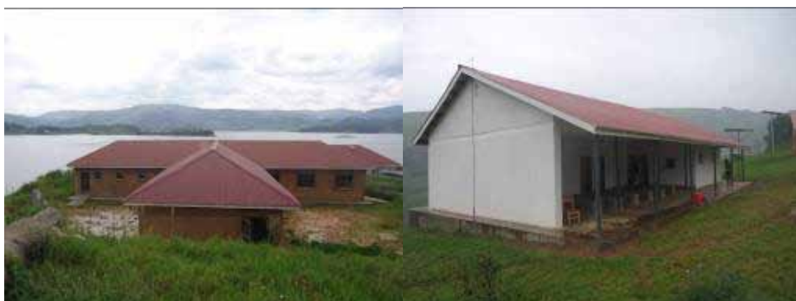
Maternity ward at Bwama HCIII and completed OPD Shebeya HCII
