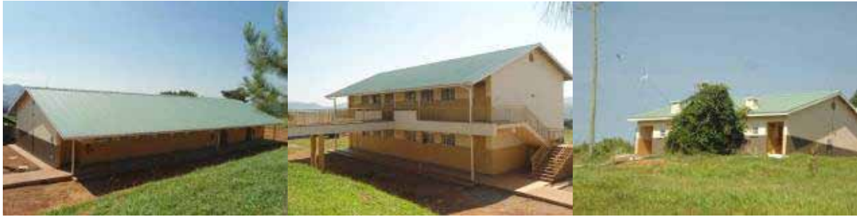
Some of the completed structures at Buhanika Seed School
