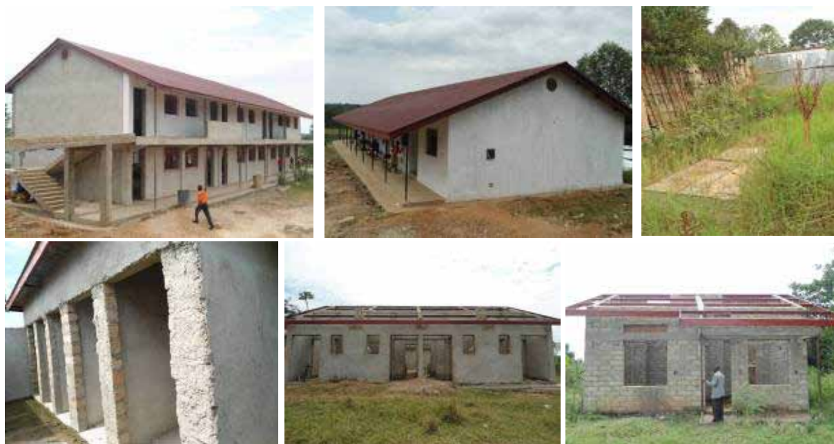
From top left, A multi purpose storied block, library with computer laboratory and a 3 stance VIP abandoned at slab level From bottom left: A stalled 5 stance VIP pit latrine, a 4 unit teachers' house and a 2 bed roomed head teachers' house that stalled at Bulamu Seed S.S.
