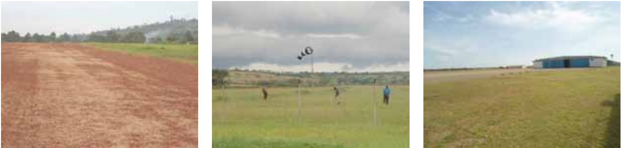
(Left): Drying weeds/grass that had been sprayed on the runway of Jinja airfield; (Centre): Slashing of the grass manually at the Mbarara Airfield; (Right): A well maintained lawn at the Soroti Airfield/Flying School.
