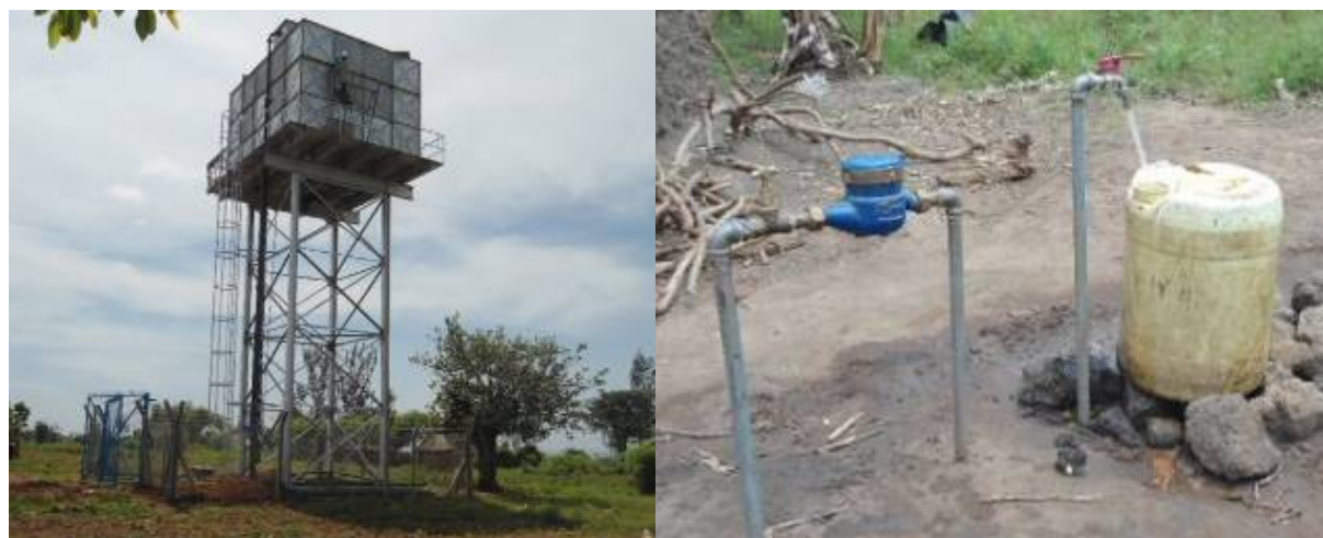
A reservoir tank with completion works ongoing and water flowing on a public tap stand as witnessed above
