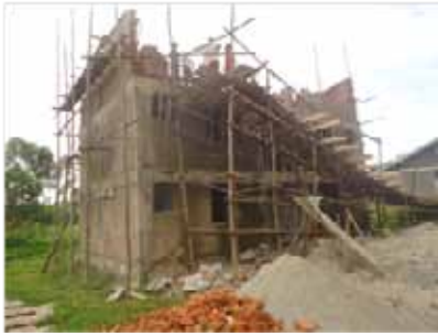
Construction of the staff house at Kataraka HCIII Fortportal Municipality.
