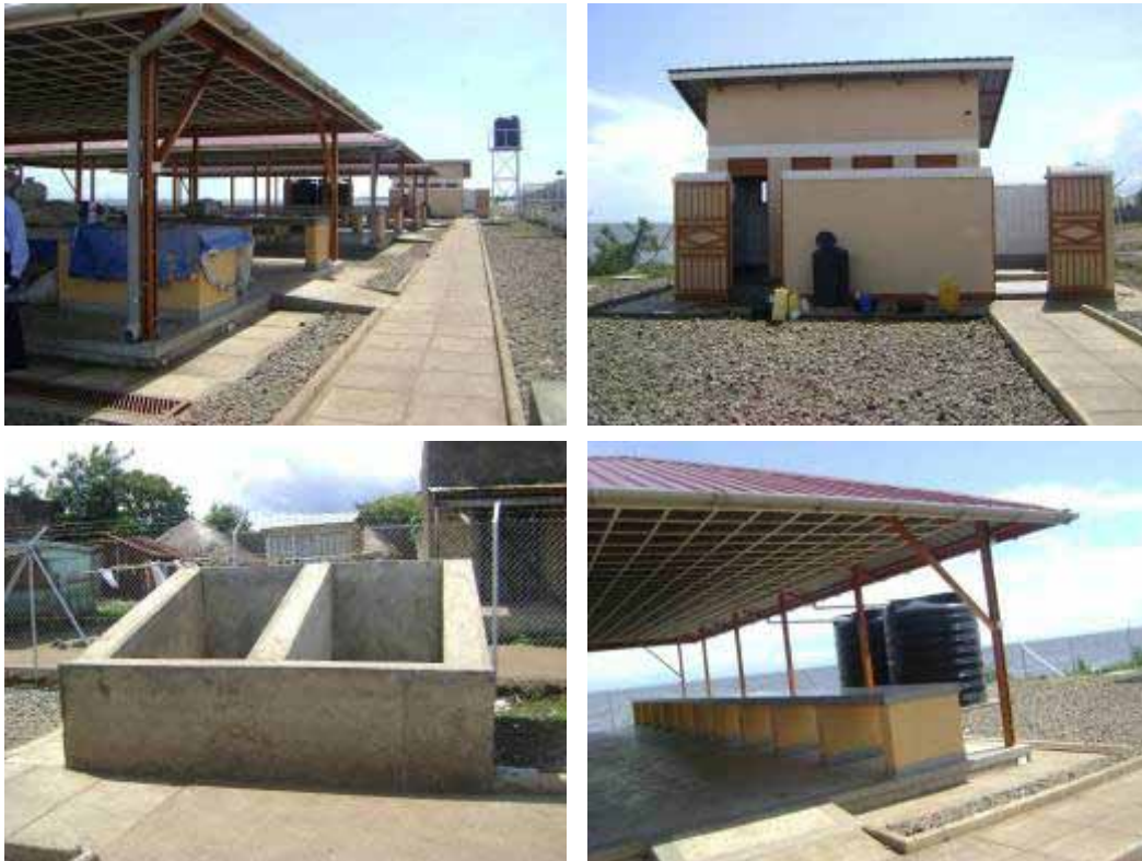
Rehabilitated Panyimur fish market in Nebbi district
