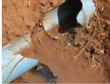
Broken pipes placed too close to the surface and not protected, Yumbe
