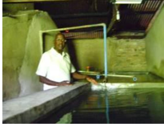
Mr. Muhoozi shows the water boiler system
