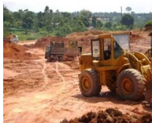
Ground leveling being done for the Kawanda substation
