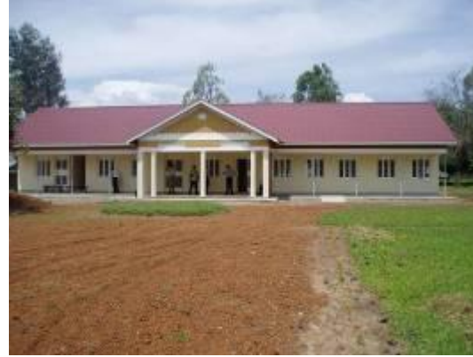
The completed administration block UCC Soroti
