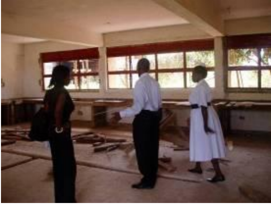
Administration block under completion at Nsambya school of Nursing
