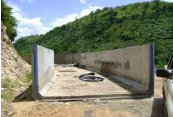
The headrace canal under construction at Mpanga
