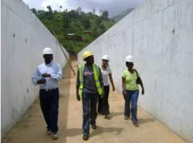
Tunnel under construction
