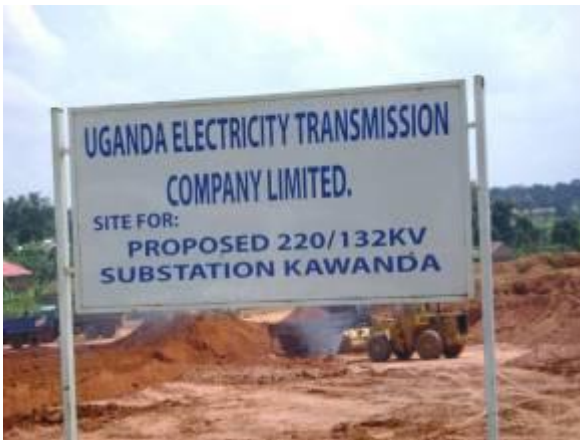
Ground leveling being done for the Kawanda substation
