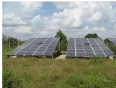
Completion of energy package, Yumbe
