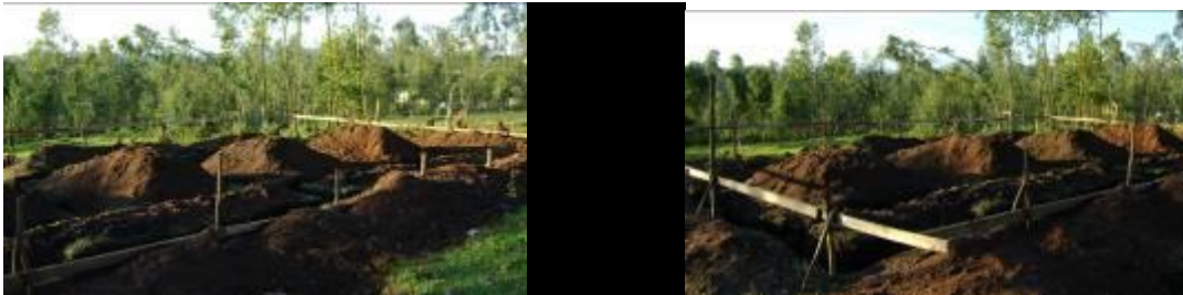
Status of Construction of Staff Houses at Kebisoni HCIV: Mid November 2008
