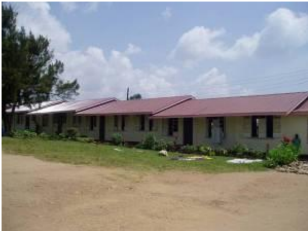
Part of the renovated dormitories at Buddo Junior
