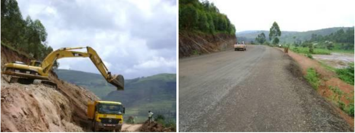
On-going earthworks and pavement construction works on Kabale – Kisoro – Bunagana road
