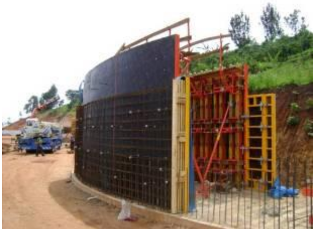
Headrace canal under construction at Bugoye power plant
