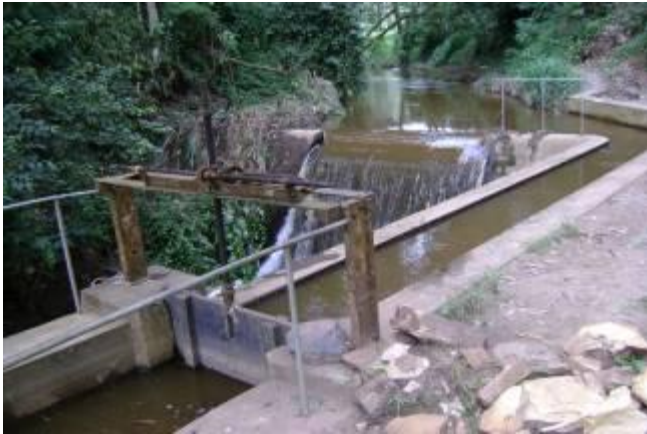
Water diversion point at Kisiizi power plant
