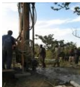
Borehole drilling by UNICEF procured contractors in Dech Sub County, Kitgum
