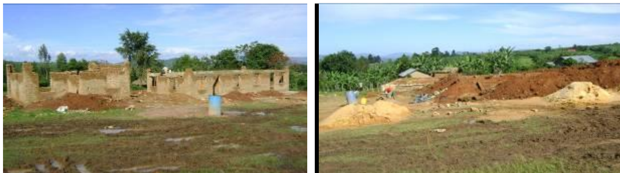
Starts of Works at Bugunga HCIV: Mid November 2008
