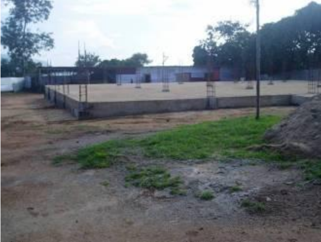
Sub Structure at UTC Elgon for the Library Block
