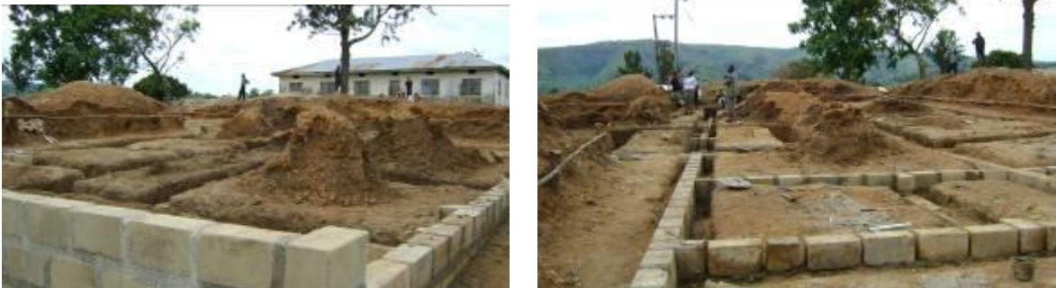
Progress of works at Shuuku HCIV: Mid November 2008
