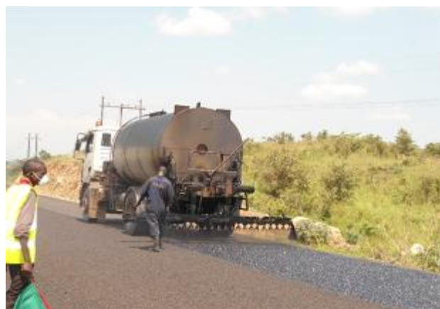
Fort-Port-Bundibugyo-Lamia road (left) excavating of the Rwenzori slopes to widen the road and to curb land slips/slides (right) priming works applied on a finished surface between Km 43+000 and Km 45+000.
