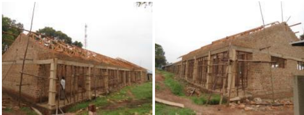
The classroom block with offices and the MV workshop at roofing level constructed at Kakiika TS
