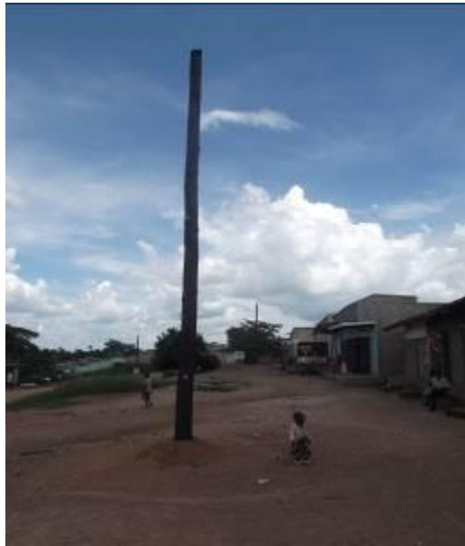
Pole erection at Ibanda-Rushere line;
