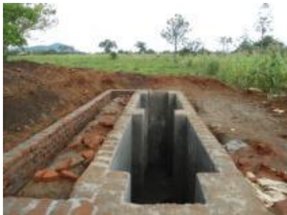
Construction of the two five-stance lined VIP pit latrines at foundation level at Kasipodo P/S
