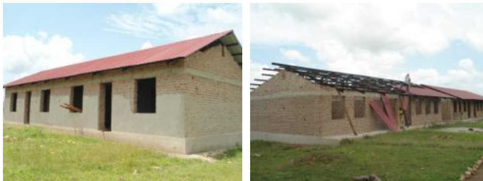
A teachers' house at finishes level and the two classroom blocks at roofing level at Kabezi Seed S.S.
