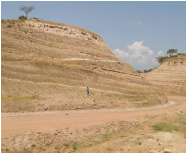
Fort Portal-Bundibugyo-Lamia road (left) A cut section and (right) A filled section on the road between Itojo and Sempaya.
