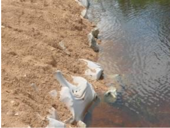
Kazo-Kamwenge road (left) Swamp treatment at Km 74+000 with rock fill and geo fabric; (right) culvert installation and area to be treated with rock fill at Km 82+823
