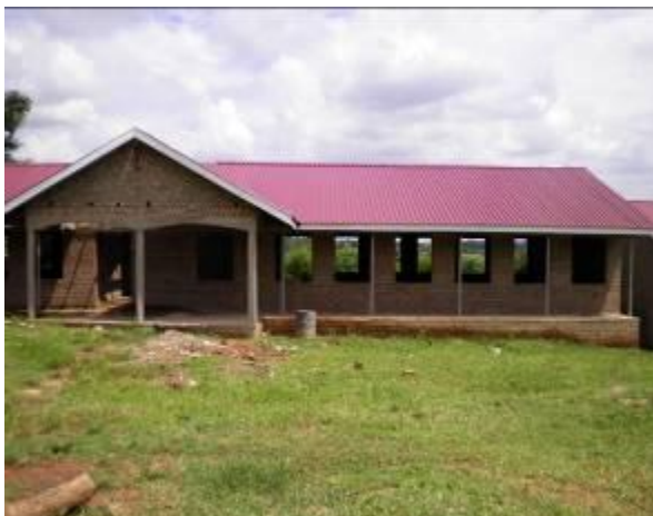
Structure at Mwererwe Secondary School
