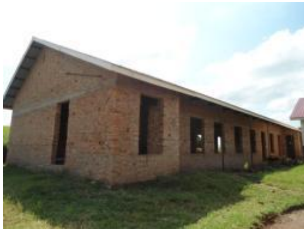
An examination hall/multi purpose hall constructed at Rubaare S.S.
