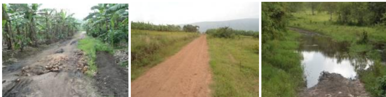
Sections of Kyazungu-Karerema road (left); Km 4+400-a section maintained by the community by putting pieces of bricks on the road(centre); at Km13+200 – graded section still in good condition. (right); Sections of Ngarama-Kigando-Kakamba road at Km7+200 with no culvert where the road was cut off.
