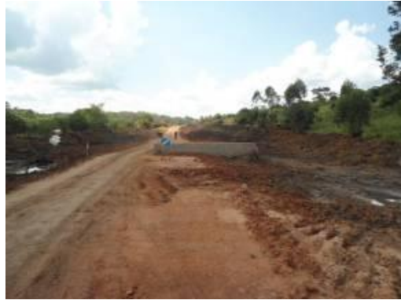
Kazo-Kamwenge road (left) Swamp treatment at Km 74+000 with rock fill and geo fabric; (right) culvert installation and area to be treated with rock fill at Km 82+823
