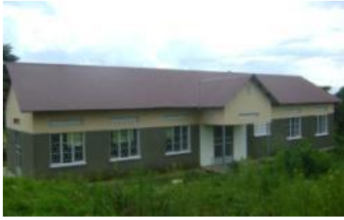
Kamwenge Local District: maternity ward at Rukunyu HCIV (above)
