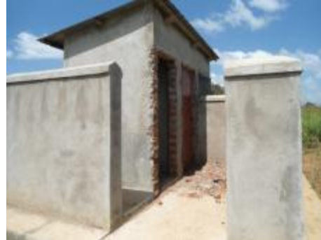
The two blocks each with two classrooms and one of the lined VIP pit latrines at finishes level at Paicho new Seed School
