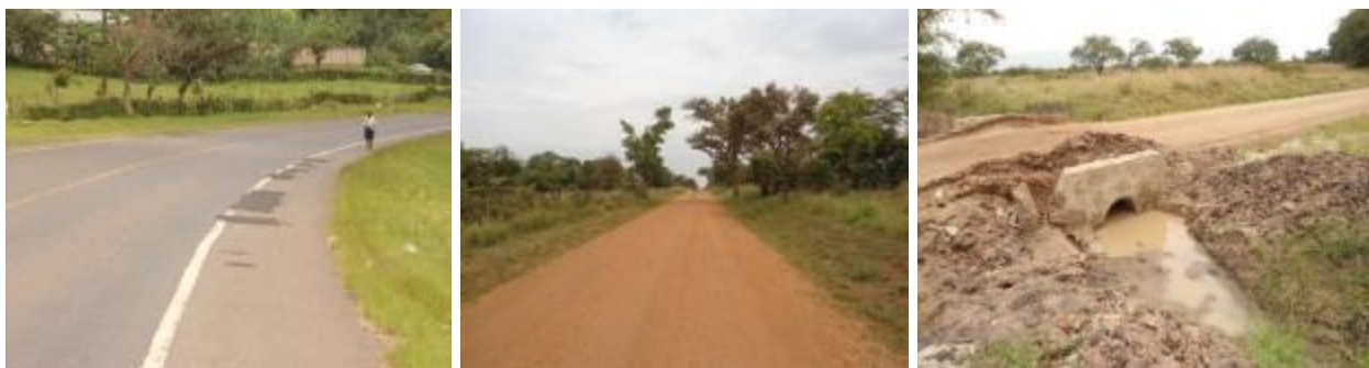
(left) Section of Fort Portal-Rwimi road which was patched with premix; (centre); Section of Karugutu-Ntoroko road graded and gravelled still in good condition; (right) Silting of culvert crossing along Kakara-Rwebisengo road.
