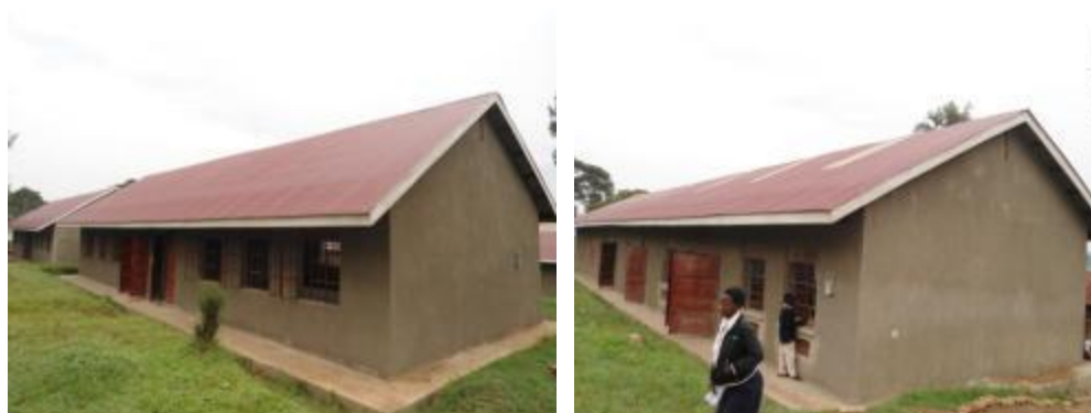
The four classrooms and the twin workshop at finishes level constructed at Kakiika TS
