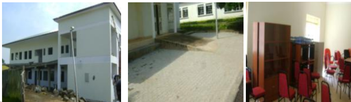
Lira Regional Referral Hospital: intensive care unit (left); paving outside information and communication centre (centre); furniture for information and communication centre
