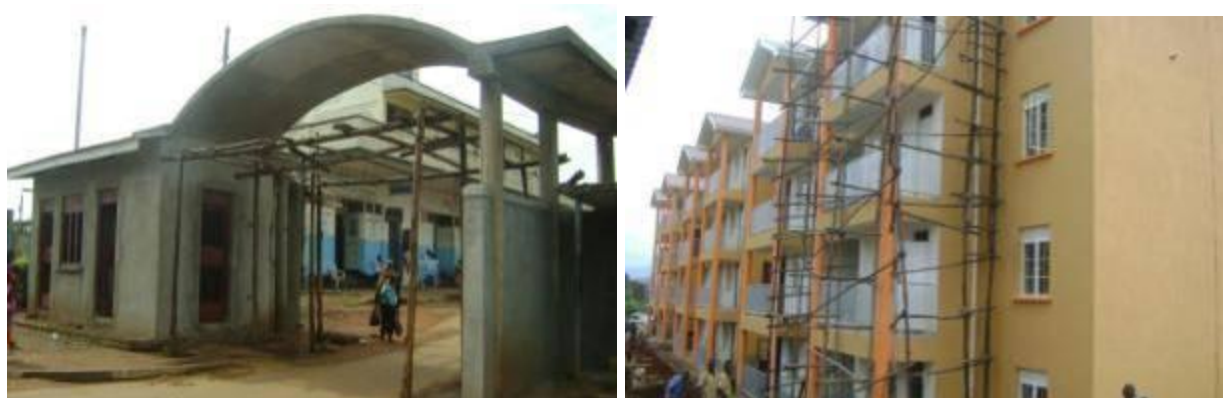
Mbale Regional Referral Hospital: hospital gate (left); senior staff accommodation (right)
