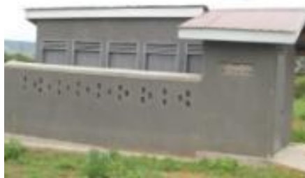
An MV workshop and a five stance VIP pit latrine constructed at Ssanje CP
