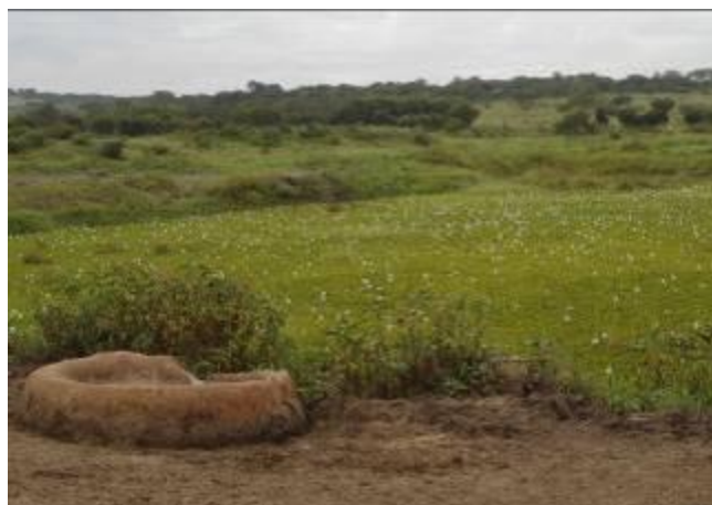
Photos: 7&8: to the left is the improvised clay cattle watering trough into which water is drawn by “shadoof” system from the dam reservoir (in background of same photo) choked up with thick vegetation. To the right is the 6m3over head tank cracked at the base and non-functional (all at Nshenyi Valley Tank Ruhama, Isingiro District.
