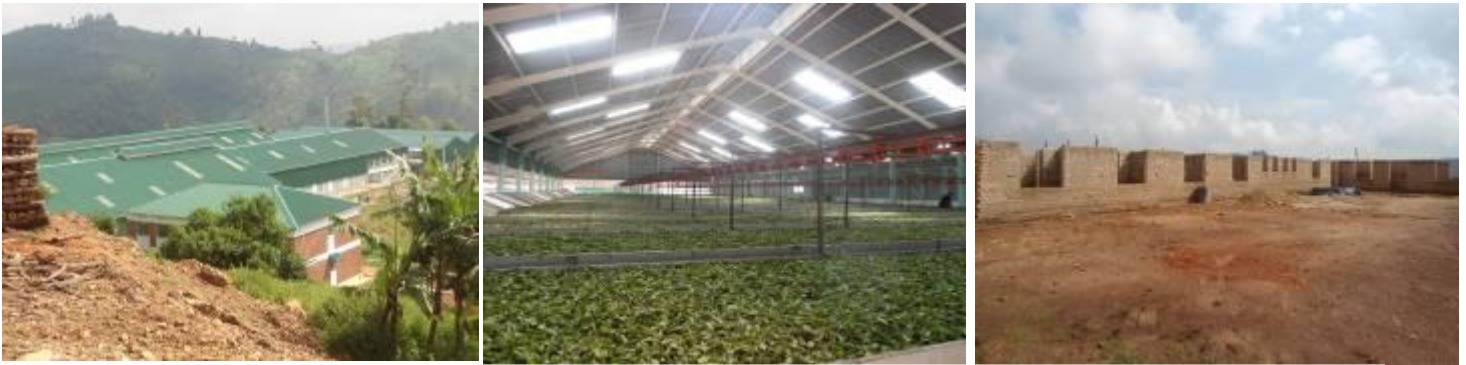
Arial view of factory complex, Tea weathering and Construction of hostel block at Buhweju
