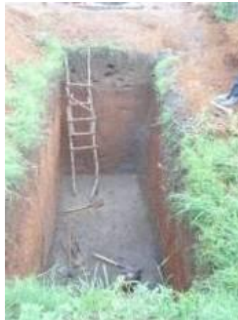
Construction of the two five-stance lined VIP pit latrines at foundation level at Kasipodo P/S
