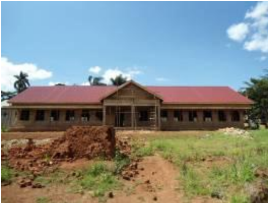
Structure at Mukono Bishop's SS
