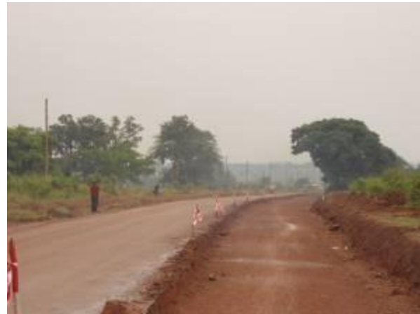
Mbale -Soroti road (left) Earth works going on along the road near. That is widening of the existing road. Notice the flat terrain in the area that has made drainage of rain water a problem slowing down the contractor.
