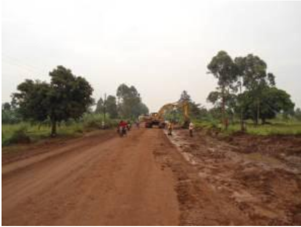
Tororo-Mbale road(left) Earth works going on along the road near Mbale. (left) Benching working going on aimed at widening of the road. Rains have hampered the contractors speed to execute works. (right) completed bench works.
