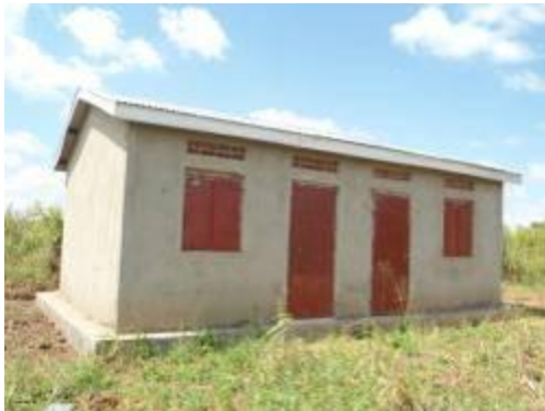
One of the two small teachers' houses constructed with savings.
