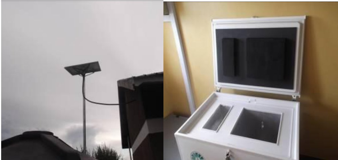
Installation of Solar panels in Mubende district; Solar fridge
