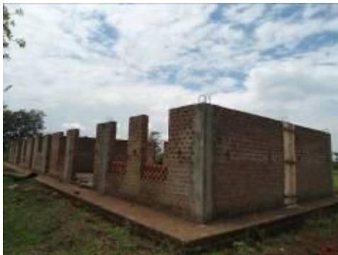
The twin workwhop for BCP and CJ at ring bim level and the kitchen shed constructed at Iyolya TS
