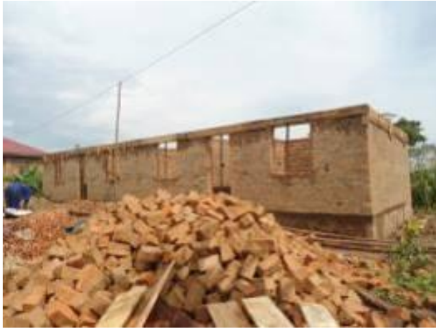
A teachers' house at ring beam level and the two VIP pit latrines at foundation level at Buwambo S.S
