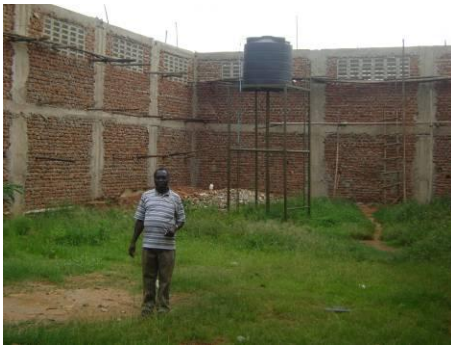
Mbale warehouse under construction
