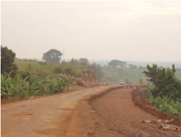
Tororo-Mbale road (left) section undergoing benching works and widening after blasting of rocks around the bend. (right) a trial section
