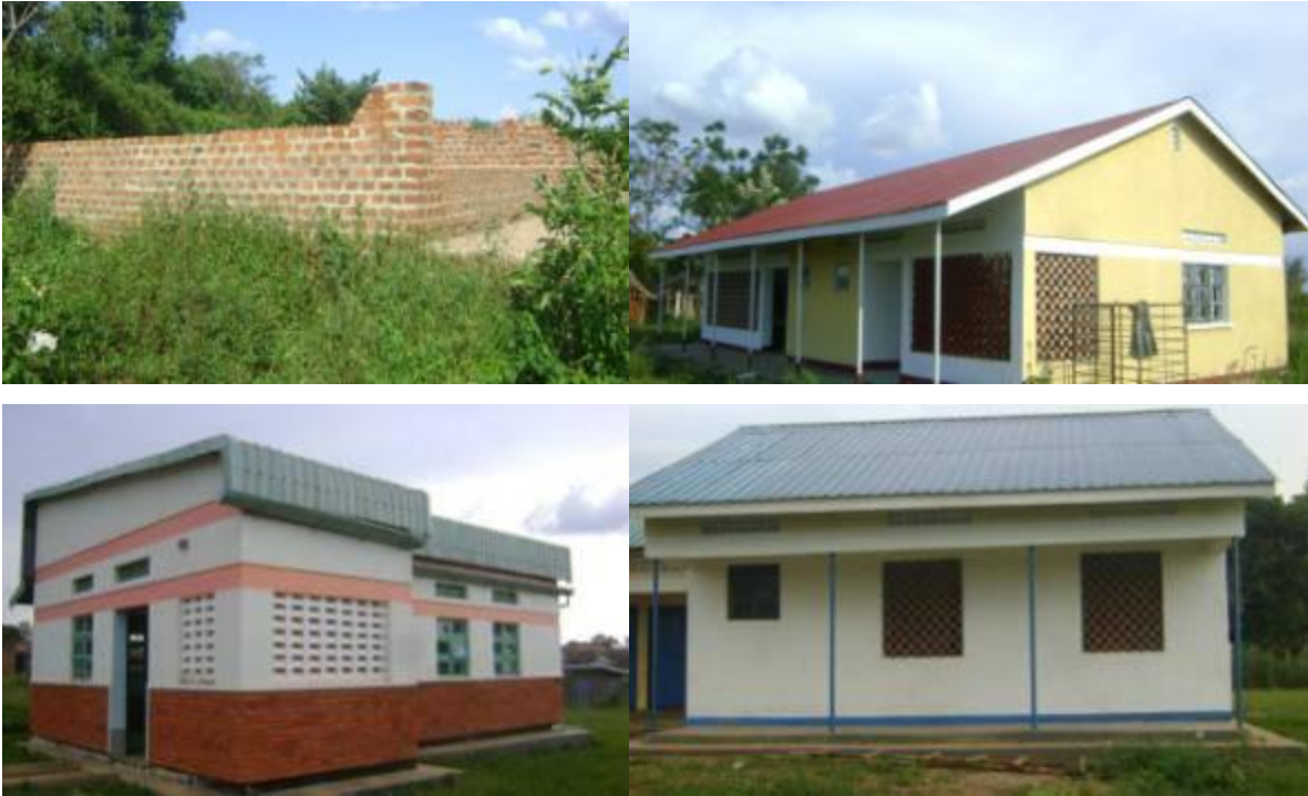
Busia District: incomplete exterior walls of OPD at Buyengo HCII (top left); staff houses at Kubo HCII (top right); laboratory at Busia HCIV (below left); extension of maternity ward at Siduka HCII(below right)
