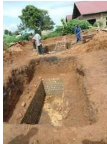
A teachers' house at ring beam level and the two VIP pit latrines at foundation level at Buwambo S.S
