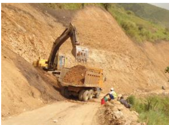
Fort-Port-Bundibugyo-Lamia road (left) excavating of the Rwenzori slopes to widen the road and to curb land slips/slides (right) priming works applied on a finished surface between Km 43+000 and Km 45+000.
