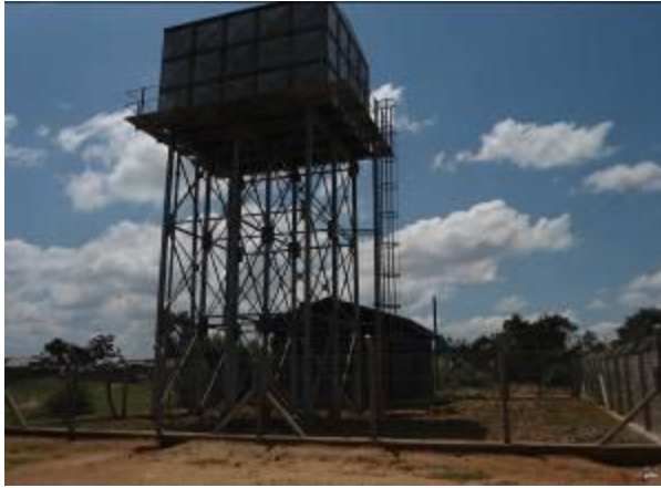
Photos 1&2: To the left is the completed reservoir Tank with the Chlorine Dosing House in the Background at Kibuku and to the Right is one of the Production Wells completed with electric cables for power to the submersible pump fitted.
