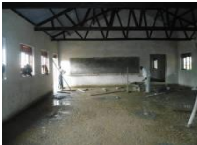
Ongoing works at St. Mary's College Rushoroza
