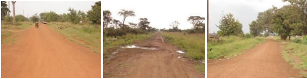
Sections of Katakwi-Usuk-Orungo (Left) Graded and graved section at Km0+000 in good condition; (Centre); failed exaction at Km 19+600; (Right) Graded and graved section at Km31+800in good condition.
