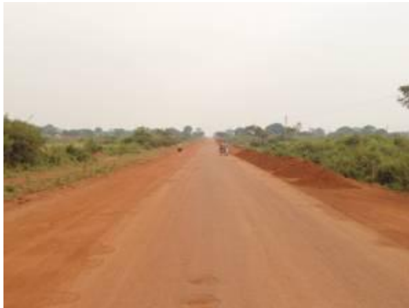
Mbale -Soroti road (left) Earth works going on along the road near. That is widening of the existing road. Notice the flat terrain in the area that has made drainage of rain water a problem slowing down the contractor.
