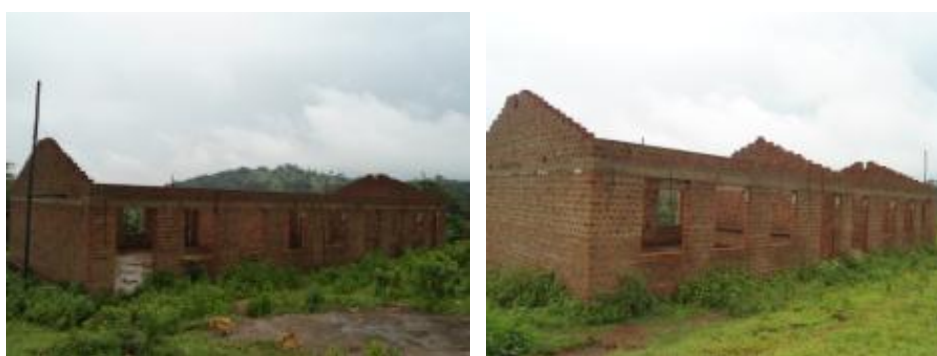
A science block and a two-classroom block at wall plate level Burunga S.S.
