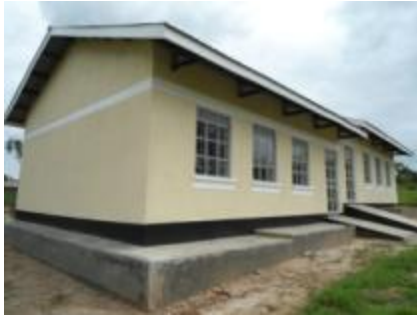
A two-classroom block completed at Ssanje CP
