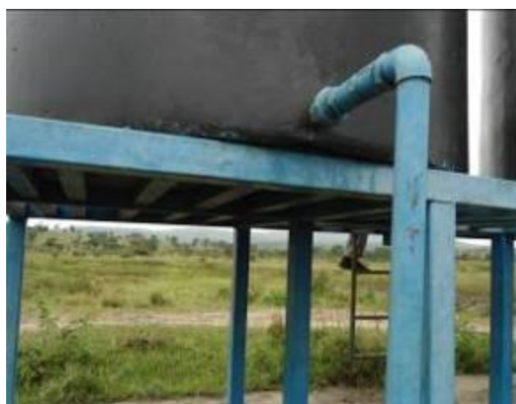
Photos: 7&8: to the left is the improvised clay cattle watering trough into which water is drawn by “shadoof” system from the dam reservoir (in background of same photo) choked up with thick vegetation. To the right is the 6m3over head tank cracked at the base and non-functional (all at Nshenyi Valley Tank Ruhama, Isingiro District.
