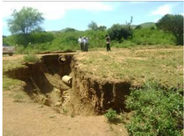
Muhokya – Kibiri road: concrete slab placed at erosion prone sections of the road (left); swept culvert and gully from an eroded culvert outlet channel
