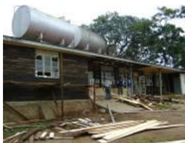
Temporary medical equipment workshop
