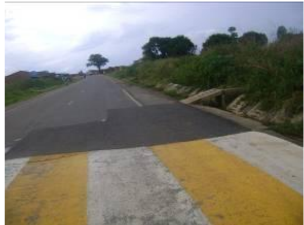
Karuma – Olwiyo – Pakwach road: Pothole patching and painting of humps
