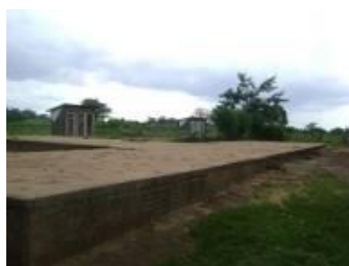
Maternity ward at foundation- Naboa HCIII
