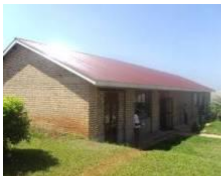
THE BIOLOGY LABORATORY WHICH WAS RENOVATED
