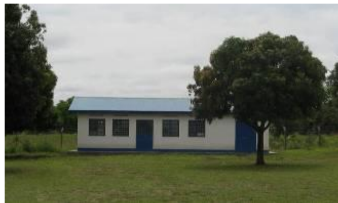
Water office constructed and ready for use, Amuria district
