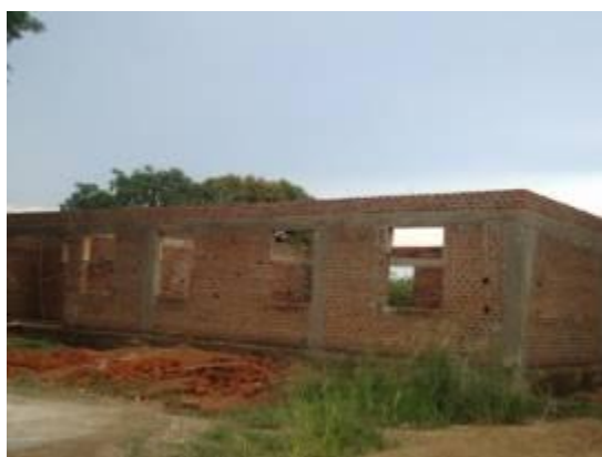
The Boys' dormitory at roofing level
