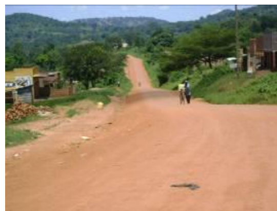
Kanoni – Maddu – R. Katonga road (60Km): a section of completed works
