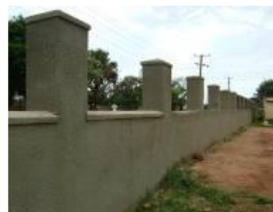
Fencing of Gulu Hospital
