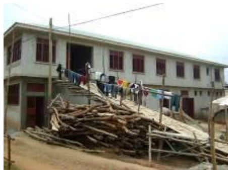
Administration and medical stores block
