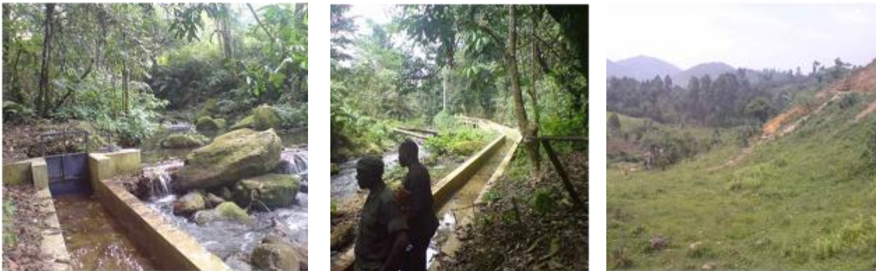
Bwindi micro hydropower project: weir; channel; site for penstock
