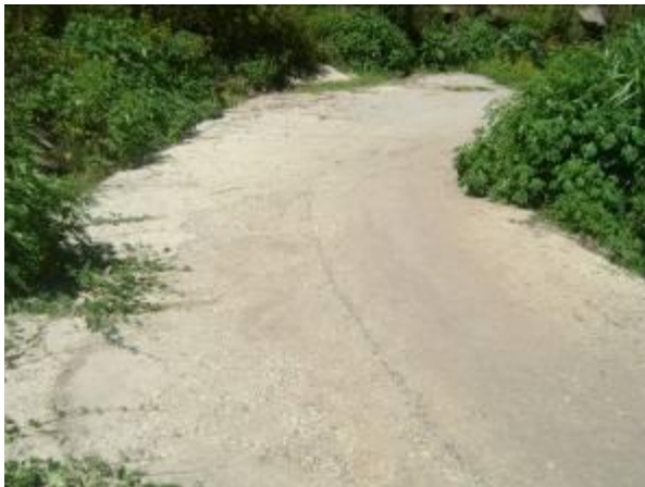
Muhokya – Kibiri road: concrete slab placed at erosion prone sections of the road (left); swept culvert and gully from an eroded culvert outlet channel
