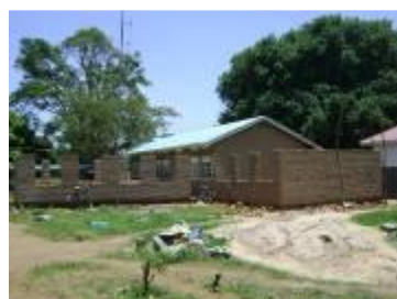
Expansion of mat. Ward Kaberamaido HCIV
