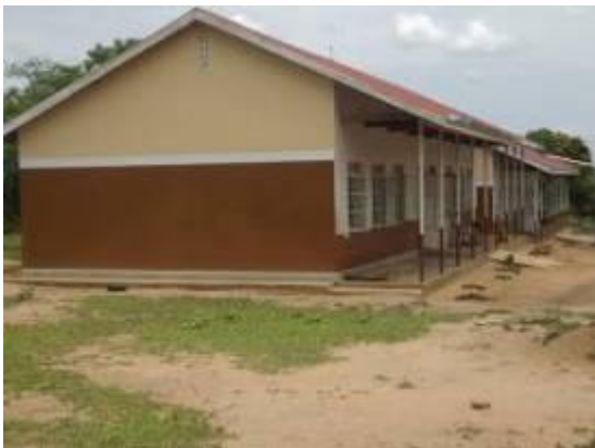
The 4 classrooms built with funding from GoU at Kinyogoga Seed S.S.
