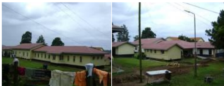
Repainted roofs of wards
