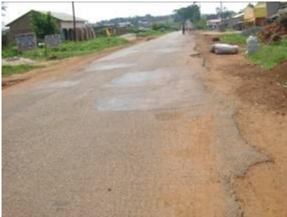
Lira –Akia road (left): pothole patching and edge failure; Lira – Aduku road (right) re-grading by force account operations.
