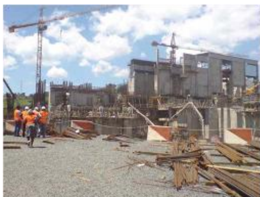
Bujagali hydropower project: construction of powerhouse; view from dam to ongoing powerhouse works.
