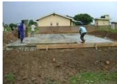
Staff house at Chaulo HCIII
