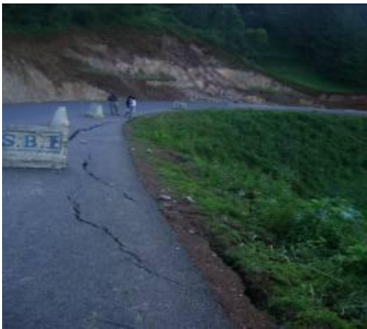
Pictures show (left) wide and very deep cracks that developed along a 100m long section of the road; and (right) collapsing side slopes that were widespread and blocking side drains at several locations along Matugga – Semutto – Kapeka road.
