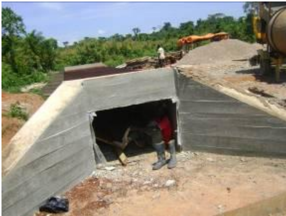
Pictures show some of the ongoing works: box culverts construction (left) and surfacing works (right) on Matugga – Semutto – Kapeka road
