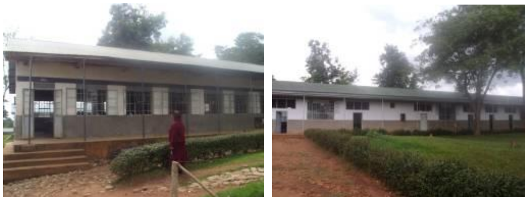
Two of the structures whose roofs were replaced at St Kalemba S.S
