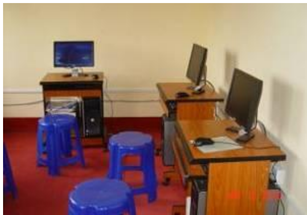
Equipment installed at Uringi S.S.S
