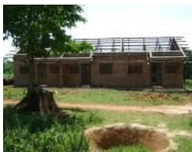
Staff house at Nawandala HCII
