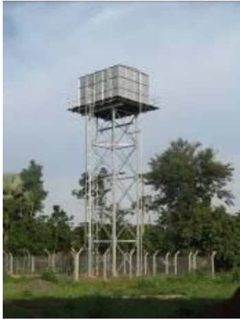
Reservoir tank constructed in Kamdini, Oyam district
