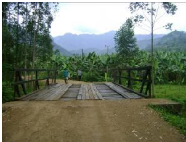
Left: Gravelled section of Mabale – Busanza (Wakamala) road; and Right: Replaced timber deck and guardrails on Bukigai – Bukalasi Bridge
