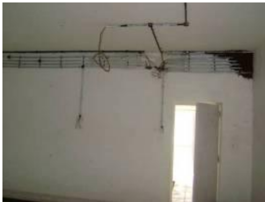
Left: Hanging electrical installations and infestation of ants in building; Right: Cracked walls of extension.
