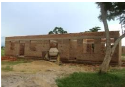
The Administration Block at roofing level
