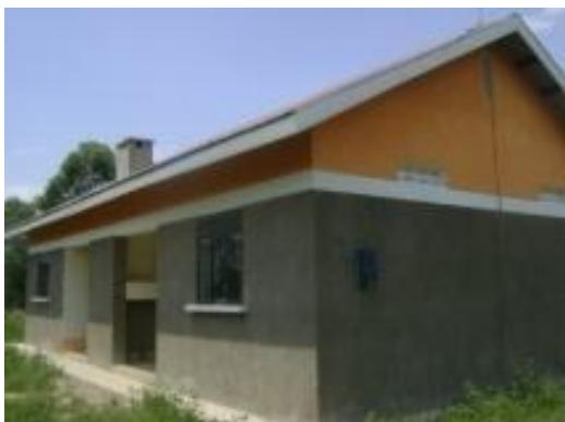
STAFF HOUSE AT KAMWENGE HCIII
