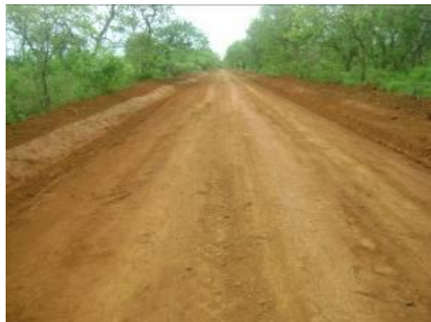
Aduku – Apire – Atar road (left): road forming by labor based techniques; and a graded section of Apac – Olelpek – Alido (right)
