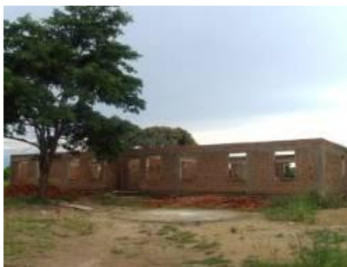
The Girls' dormitory at roofing level
