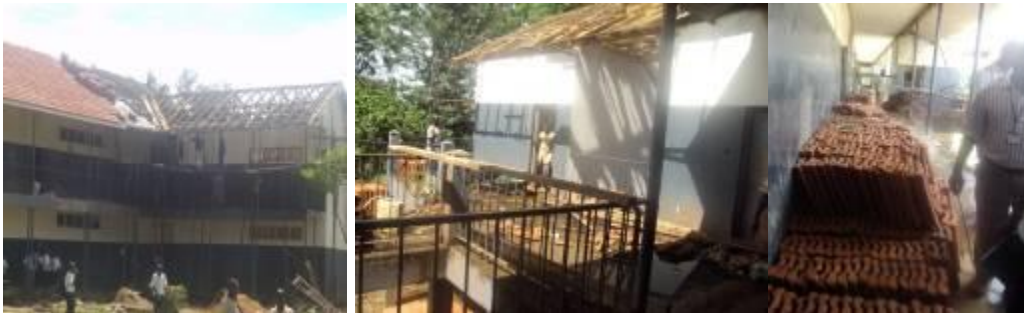
The ‘A’ level block housing 18 classrooms being renovated at Jinja S.S.
