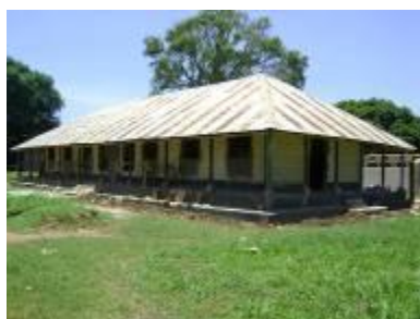
Rehabilitation of Gen ward, Kaberamaido HCIV
