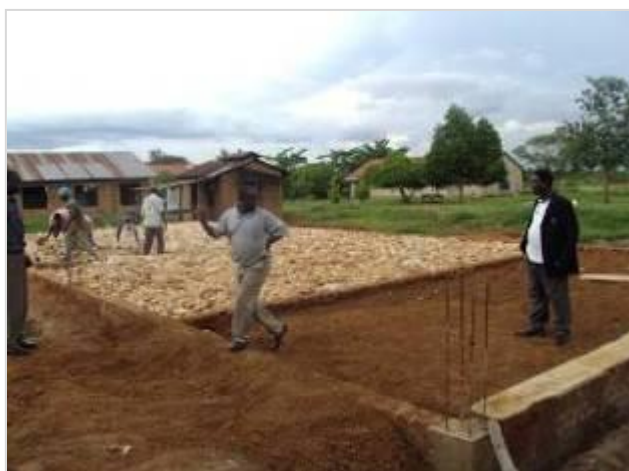
The Dining Hall at foundation level
