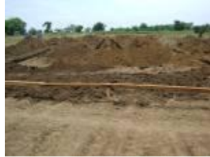
Excavation for DHO's office
