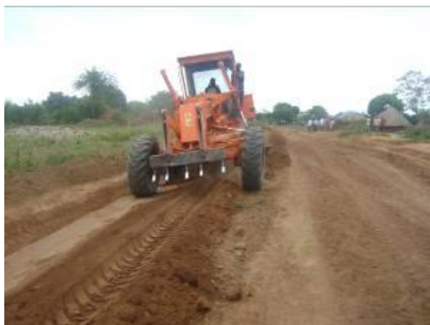
Grading in progress on Kabukol – Kamenya road (left) and a section of completed works on Kumi – Malera roads
