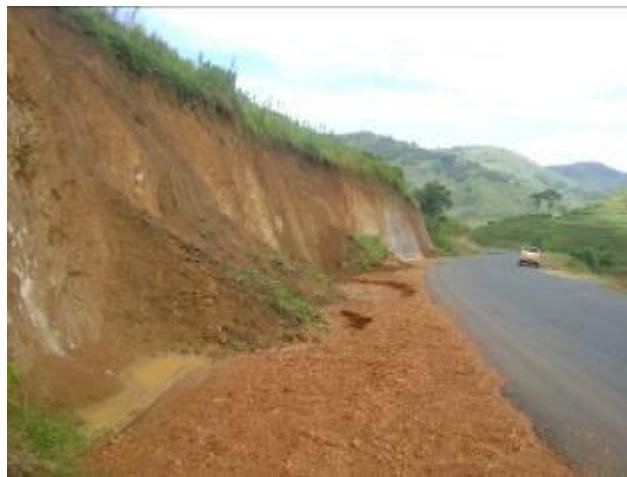
Pictures show (left) wide and very deep cracks that developed along a 100m long section of the road; and (right) collapsing side slopes that were widespread and blocking side drains at several locations along Matugga – Semutto – Kapeka road.
