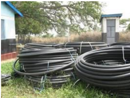
Pipes delivered for extension, Moroto district
