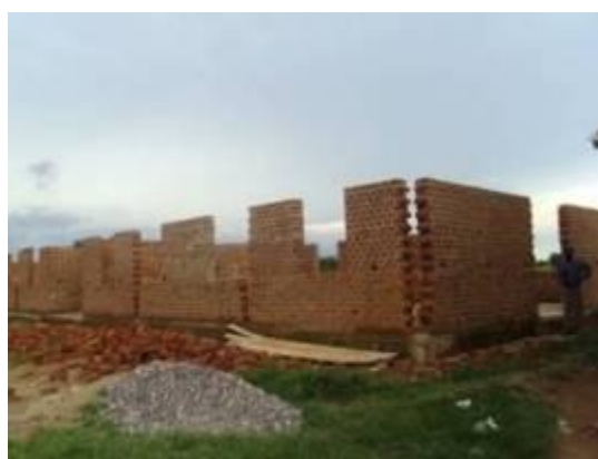
The CJ workshop at ring beam level
