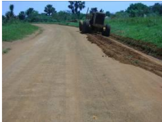
Lira –Akia road (left): pothole patching and edge failure; Lira – Aduku road (right) re-grading by force account operations.
