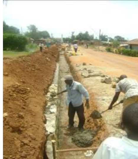
Naboa Street reportedly complete but poorly surfaced (left); and construction of stone lined side drains in progress on Gangama road
