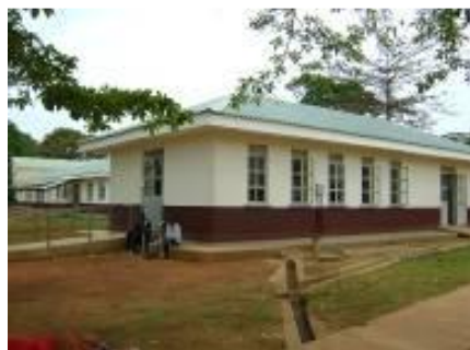
Medical ward completed & in use
