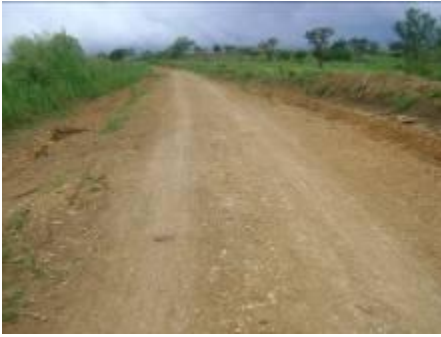
A section of completed works in Section A of the road
