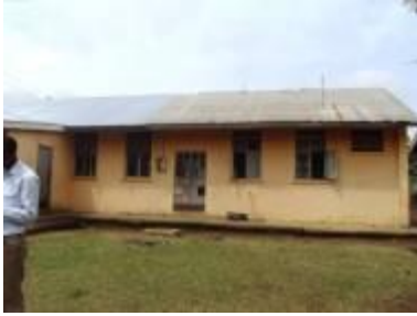
The Home Economics Laboratory at Ngora Girls before the renovations
