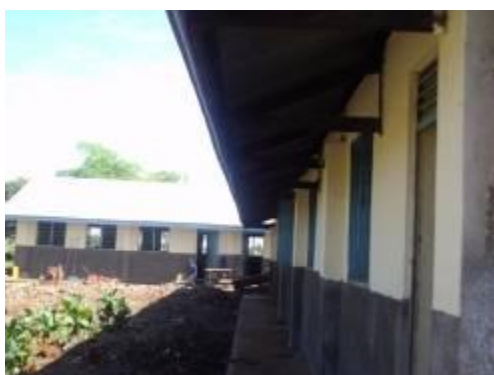
The 4 classrooms which were renovated
