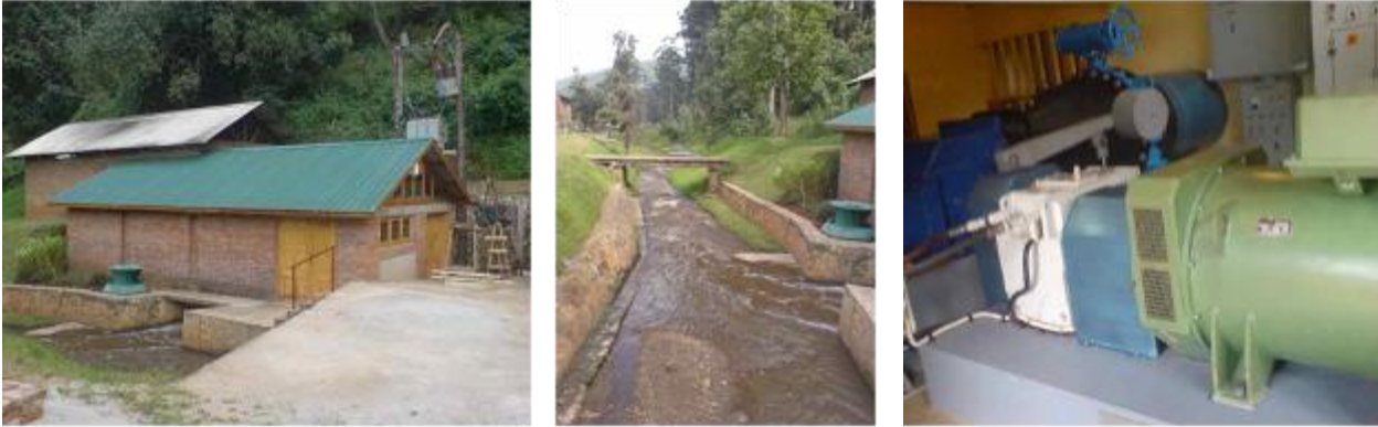
Kisiizi micro hydropower project: completed powerhouse; channel; new generator
