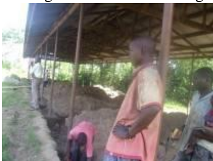
A 2 classroom block being constructed at Bundikahunga P/S
