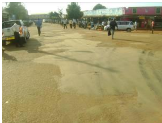
A section of the road bed of Tensing Road (left): and excessive bleeding of newly constructed asphalt patches on Bazaar Street (right)
