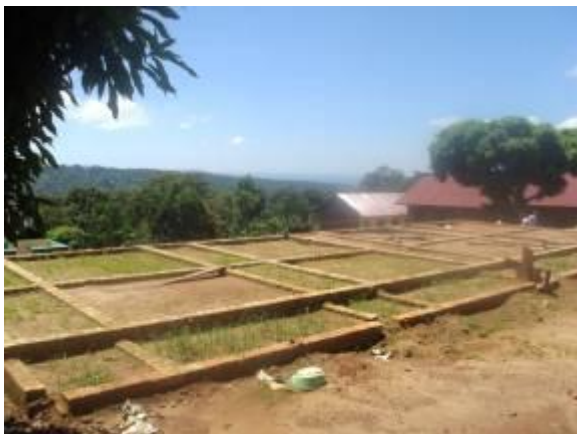
The foundation for the 4 teachers' houses that had stalled.
