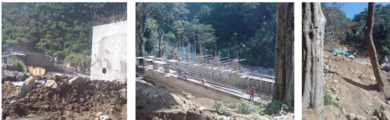
Mpanga hydro-electric plant: dam construction; powerhouse (rear view); site for penstock.
