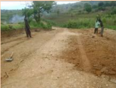
Drainage works in progress in section B of the road
