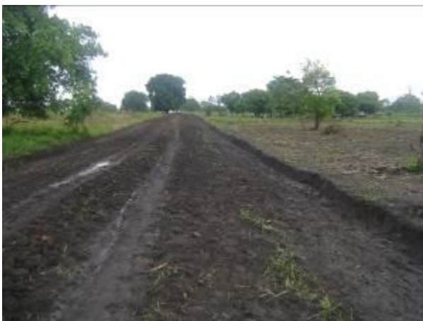
Aduku – Apire – Atar road (left): road forming by labor based techniques; and a graded section of Apac – Olelpek – Alido (right)
