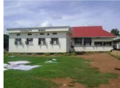
Causality ward renovated
