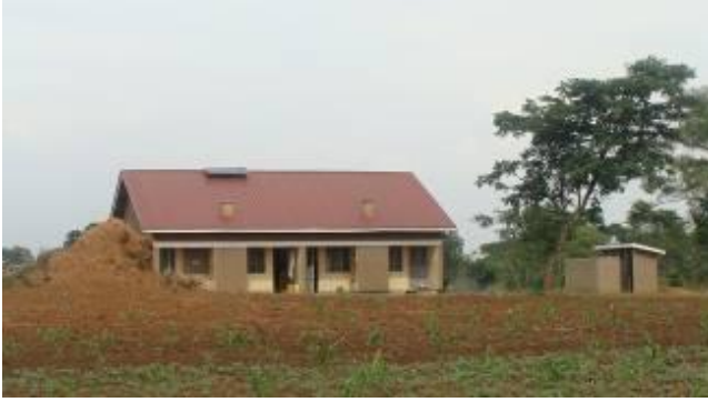
Staff house in Namusaala Kayunga District powered by EAP solar system
