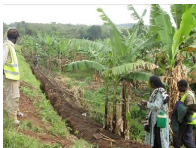
Supervision of works at Hima RGC, Kasese district
