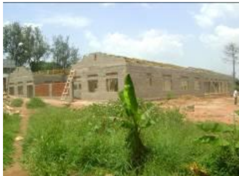
Mental health unit at roofing stage
