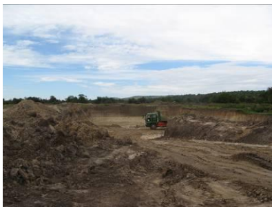
Works ongoing, Obwengyerero Valley Tank
