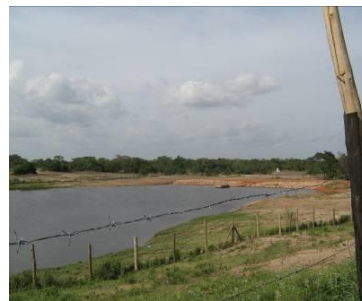
Bwanalaki dam near completion
