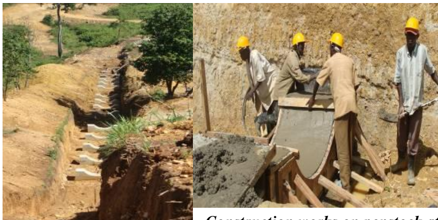
Construction works on penstock at Ishasa
