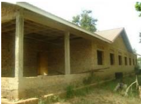
Construction of OPD at Nakasongola HCIV
