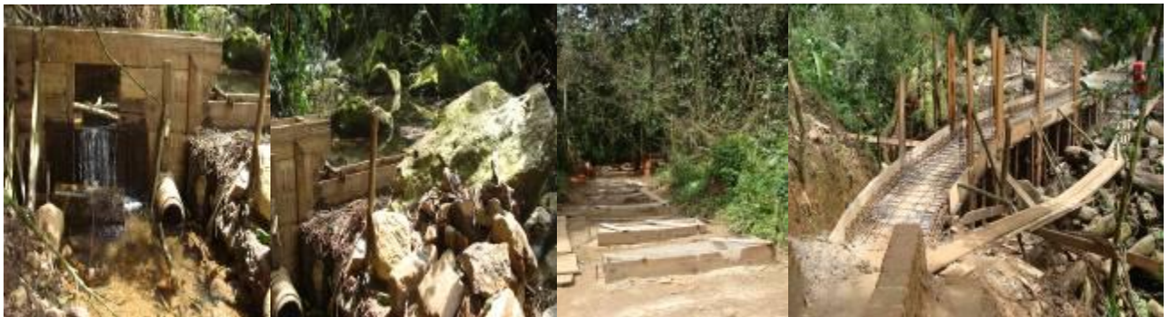
Construction works in progress at Bwindi mini HEP
