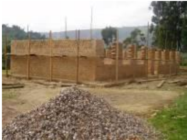
Construction at Kitagata Farm School
