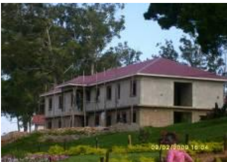
Private ward under construction
