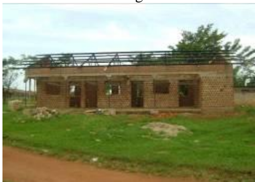
Construction of OPD at Ntwetwe HCIV
