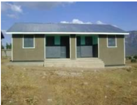
Staff house constructed at Iri HC III
