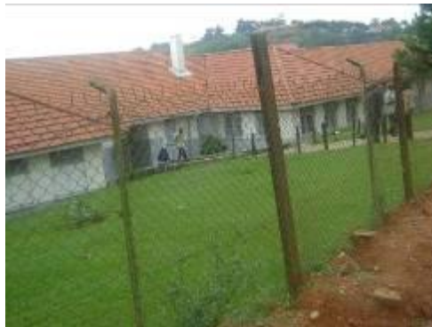
Maternity ward after rehabilitation
