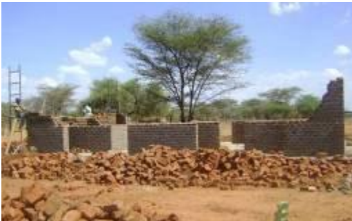
Staff house under construction at Nadunget
