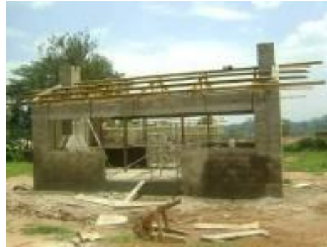
Laundry at roofing stage
