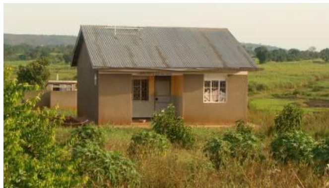
Busegula Health Unit staff house with missing solar panels.
