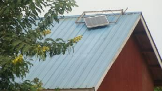
Dismantled solar panels on Namusaala HC OPD
