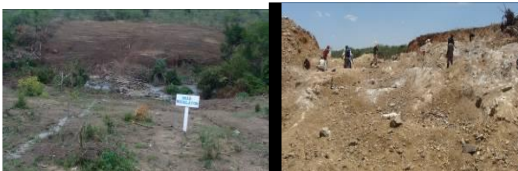
Construction works on Buseruka dam and blasting works on canal path.
