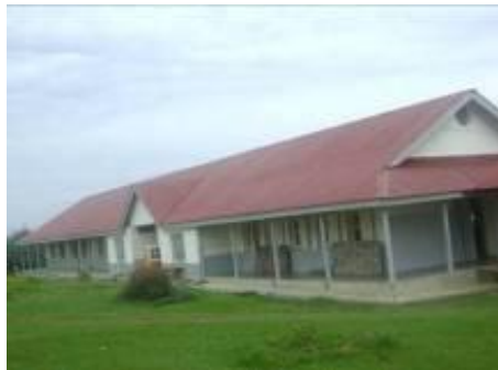
Rehabilitated Tuberculosis ward
