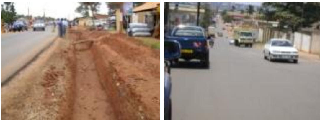
Pictures show ongoing drainage works with a weak shoulder/ drain interface on Ntinda – Kisaasi road and completed works on Kibira road.
