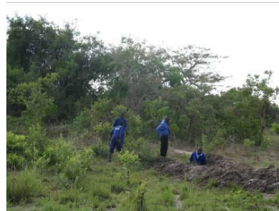
NWSC working on broken pipeline
