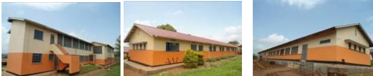
Mayanja, Nkoyoyo and Nassolo dormitories renovated at Nkoyoyo Boarding P/S
