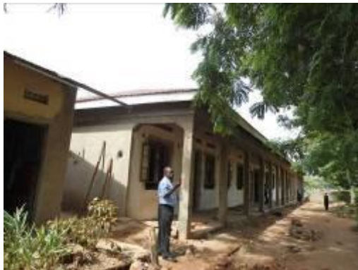
A rehabilitated library block at Namagabi S.S
