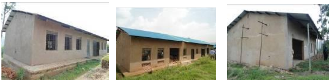
A BCP & CJ workshop, a 2 classroom block and an MV workshop constructed at Rukore CP
