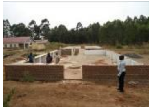
A dormitory block at window level at Arua T/I
