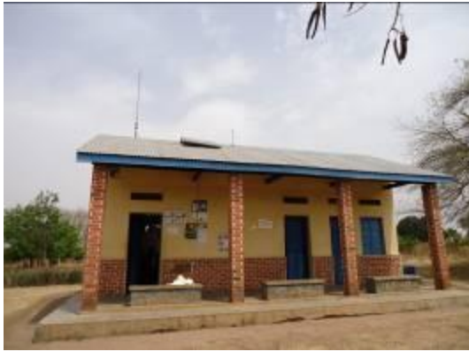
L-R: Solar installation at Munu HCII District
