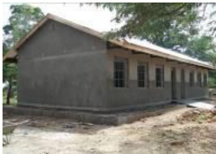
A2 classroom block at finishes level at Namutumba P/S
