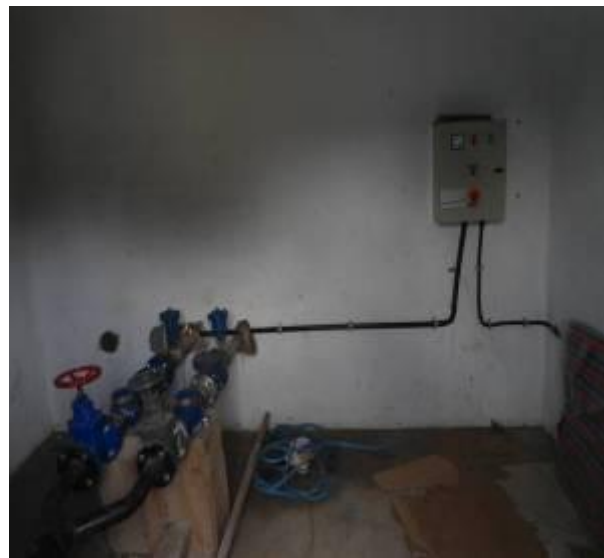
Pump house and Control Room (Left) and interior of the Control Room (Right) for Nakaseke Town Water supply and Sanitation System. The site is in a marshy area and floods during heavy rains. This is likely to cause costly problem in future. (07/03/2012)
