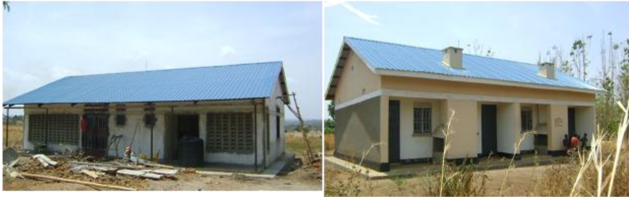
Yumbe District Local Government; OPD at Gitara (left) and staff house at Al-noor HCII
