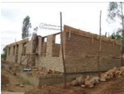
The administration block at ring bim level and the dormitory block at wall plinth level at Karera T/I
