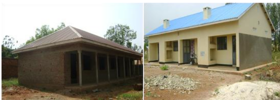
Gulu municipal council; stalled office block health department (left) and completed staff house at Laroo HCIII (right)
