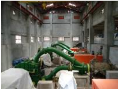
L-R: The 3x3MW turbines installed in power house. Dam section under construction. Fore bay at Buseruka HEP
