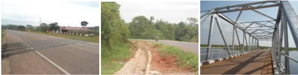
(Left): Section of Gayaza-Kalgi road with rumble strips near Naigaga market (Centre): Stone pitching at Nakifuma along Kalagi-Kayunga road. (Right): Painting of trusses, railing and kerblines of Sezibwa bridge along Kalagi-Kayunga road.
