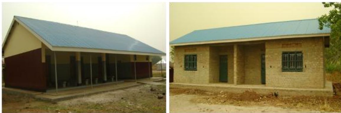
Oyam District Local Government; OPD at Iceme HCIII (left) and semi-detached staff house at Agulurude HCII (right)
