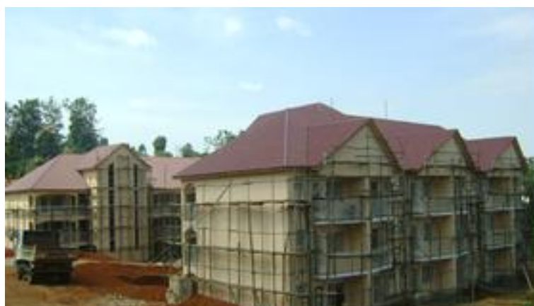
Masaka Regional Referral Hospital; staff hostels under construction
