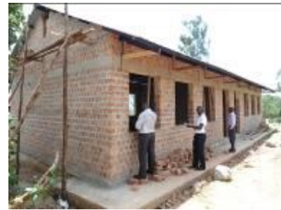
A 2classroom block at Kasengejje P/S
