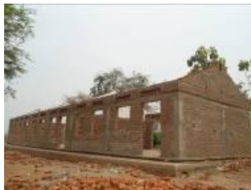
A 3 classroom block constructed at Inde T/S
